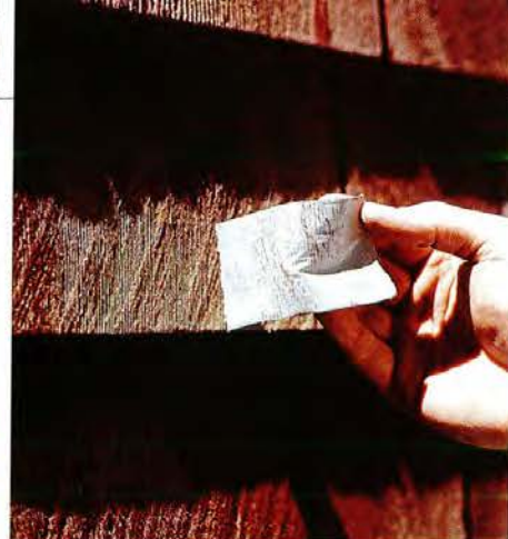
LEFT: Painter Seth Knipe blasts away weathered paint and wood to restore a sound surface to the shingles on an old barn. ABOVE: A piece of duct tape shows how the sun has loosened surface fibers of the wood.
