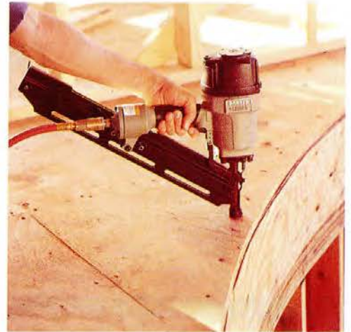
FC350 Framing Nailer-Clipped Head - Use for all framing jobs including subflooring and wall sheathing.
