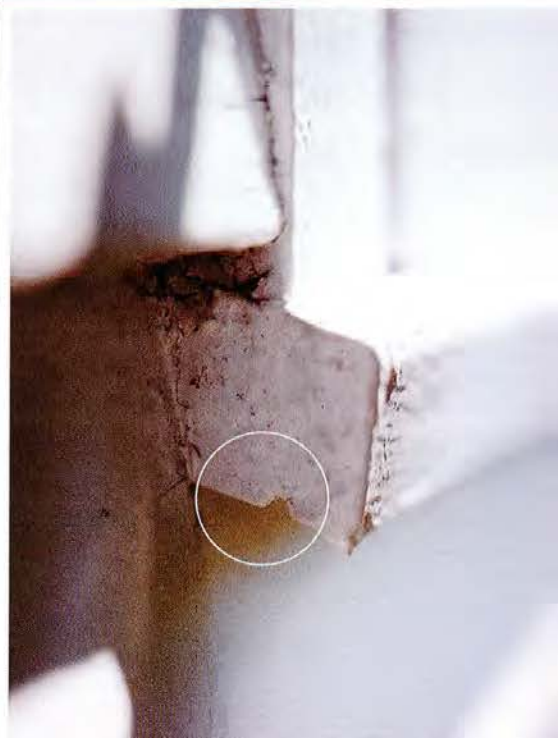
TOP: Good gutter screens let in water, keep out leaves and swing out of the way for routine maintenance. ABOVE: With a fresh application of mortar, a repointed brick wall is like new. RIGHT: The drip groove kerfed into the bottom of this window-sill stops water from finding its way behind the siding.
