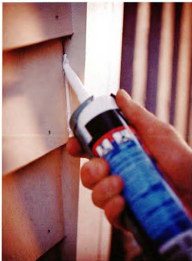
TOP: A foil-covered foam box, dogged down with straps, minimizes the heat loss through normally leaky attic hatchways. Loosen the straps, and the lightweight box moves aside for attic access. ABOVE: A paintable silicone sealant keeps air from finding its way between clapboard and corner board.
