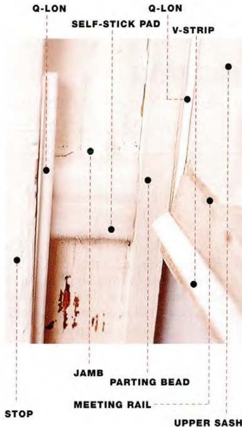
LEFT: A drafty double-hung window becomes almost as tight as a new one with some strategically placed weather stripping. Q-lon stapled to the stop and parting bead seals the sides of the sash. The V-strip goes across the meeting rail, the bottom of the lower sash and the top of the upper sash. The self-stick pad stops air from sneaking in through the jamb. ABOVE: Ceiling penetrations around old pipes and wiring deserve a shot of canned foam, the button-upper's best friend. BELOW: A router plows the groove for an adjustable door sweep that stays out of sight.
