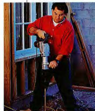
Ron Miller drives a 10-foot ground rod at least 2 feet from an exterior wall, above, and then attaches the cable to the rod, below.
