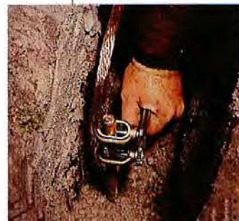
Ron Miller drives a 10-foot ground rod at least 2 feet from an exterior wall, above, and then attaches the cable to the rod, below.
