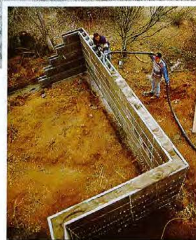
RIGHT: To enclose the new master-bedroom suite, the crew built walls of polystyrene blocks and pumped them full of concrete grout. ABOVE: A crenellation at the top corner of the suite was added to mimic the way real adobe degrades from exposure to wet weather.
