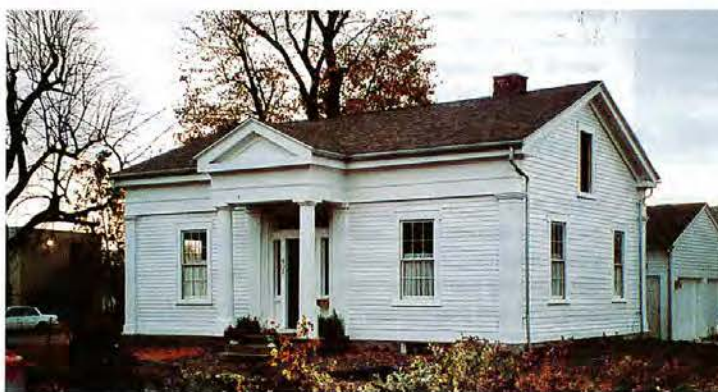
After removing the old paint with a rotary grinder, Michael Hunt coated the wood with a water-repellent preservative, then a latex primer. He finished up with two coats of latex paint. Five years later, there is still not a flake in sight.
