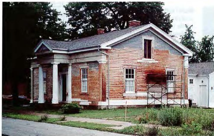
When Michael O. and Phyllis J. Hunt bought this 1858 Greek Revival in Lafayette, Indiana, they ripped off asbestos shingles and found thickly painted yellow poplar underneath. Michael, who runs the wood research program at Purdue University, followed the advice of the Forest Products Laboratory and restored the old siding with new paint.
