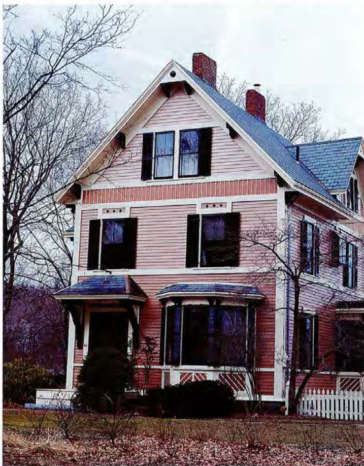
When a paint job costs $40,000—as it did on this 5,529-square-foot Victorian in Concord, Massachusetts—you just pray it lasts. The walls and trim were scraped to bare wood, primed and coated with two layers of oil paint imported from Europe.
