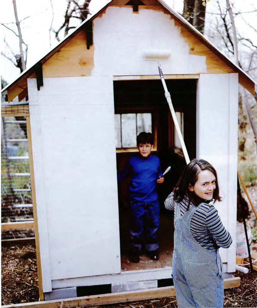
Jake DeMichele supervises as Olivia Carrano finishes painting the coop's half-inch plywood siding. Salvaged windows bring in light, and triangular openings in the eaves provide ventilation.
