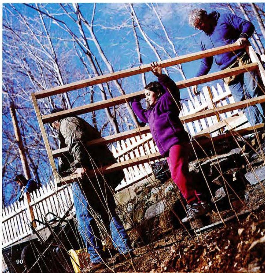
Ten-year-old Olivia Carrano—stationed behind her father, Robert Carrano, and in front of carpentry teacher Mark DeMichele—helps hoist a wall section. Because the coop is built on a steep slope, they assembled the frame on the flat driveway, then carried it to the site.
