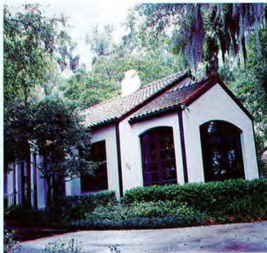
Bill and Sandy Kirk expect to cut the monthly cost of cooling their 1,800-square-foot house in Winter Park, Florida, from $220 to $145.
