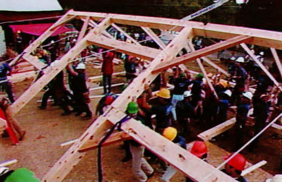
ABOVE: With pike poles and muscle, students of post-and-beam construction raise the frame, just as neighbors must have helped haul up the original. OPPOSITE: The view from the view. It was the prospect of looking out at this pond that got the Wickwires thinking about living in their barn.
