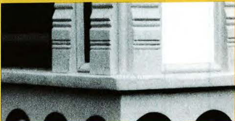
...sanded, nailed, stained or painted.
