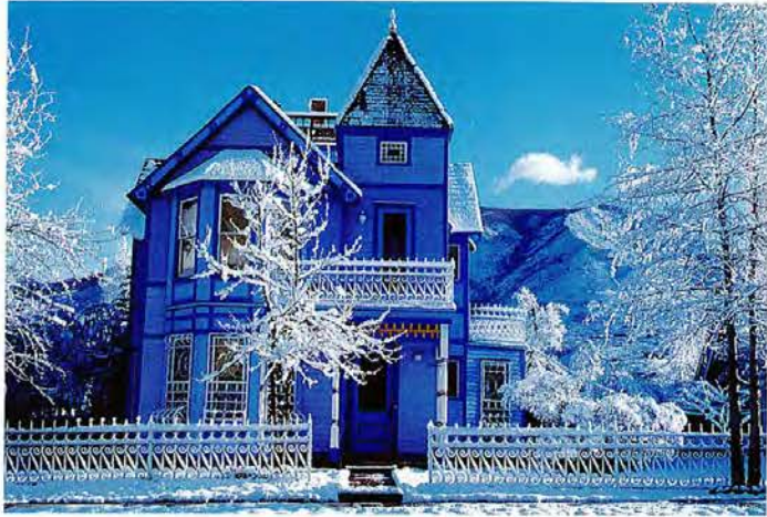
ASPEN, COLORADO: Elaborate ironwork, mass-produced in Victorian-era factories, gave character to the simplest houses.
