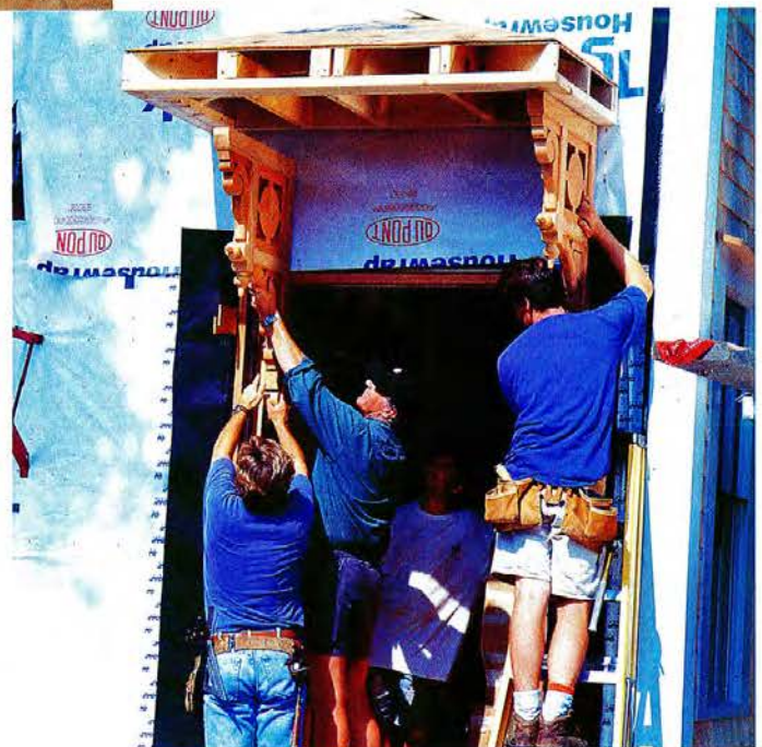
LEFT: Easing the edges with sandpaper, Norm Abram finishes one of four brackets he built from mahogany and recycled cypress. BELOW: With the portico roof in place, Steve Thomas, Bruce Killen and crew members hoist the brackets for the front entry.
