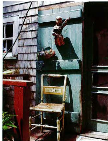
An open batten door on The Little Red House reveals the ledge boards that hold it together.
