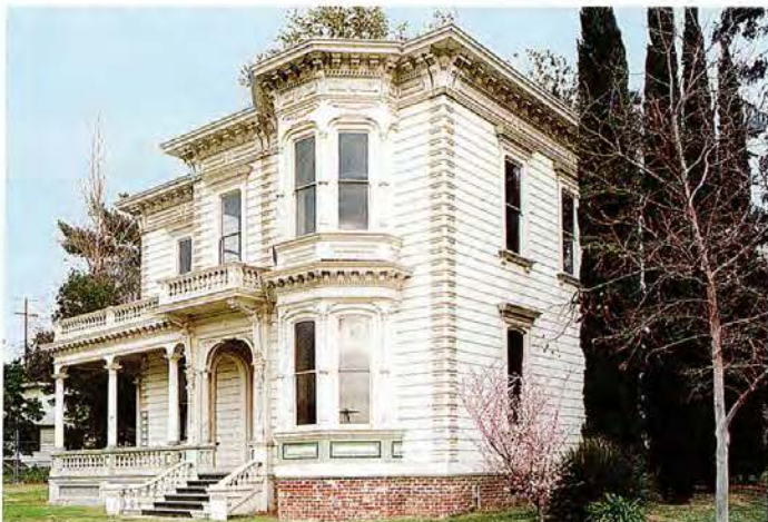
LOS ANGELES, CALIFORNIA: As if zippered with cut stone, this Italianate's quoins are all illusion: Victorians used wood to replicate anything they saw in classic stonework.
