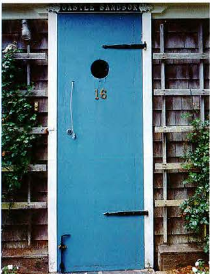
From an era with fewer security concerns, a rope pull lifts the latch inside this 1814 door.
