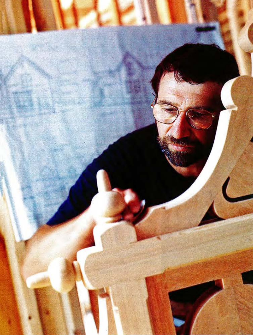
LEFT: Easing the edges with sandpaper, Norm Abram finishes one of four brackets he built from mahogany and recycled cypress. BELOW: With the portico roof in place, Steve Thomas, Bruce Killen and crew members hoist the brackets for the front entry.
