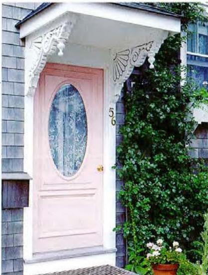
Like 19th-century Victorian details, brackets for this 1991 house came from a catalog.
