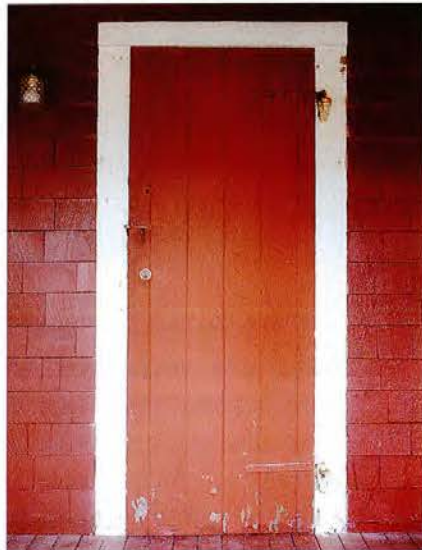
The essence of simplicity: strap hinges, a latch and no doorknob.
