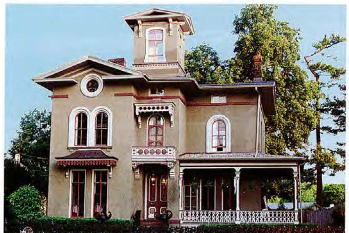
FRENCHTOWN, NEW JERSEY: Add a tower and smooth stucco walls, and an Italianate becomes a Villa style. Towers were vestigial lookouts, often unused and even unfinished inside.
