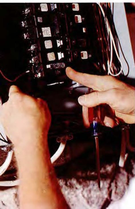
BREAKER PANEL PHOTOGRAPH BY KELLER & KELLER; GFCI OUTLET BY DARRIN HADDAD
