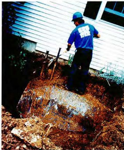
Doug Lawless, a technician for a New Jersey environmental cleanup company, shovels dirt from the fill and vent pipes of a tank in Clinton, New Jersey. Power equipment might break the pipes, allowing oil to spill.
