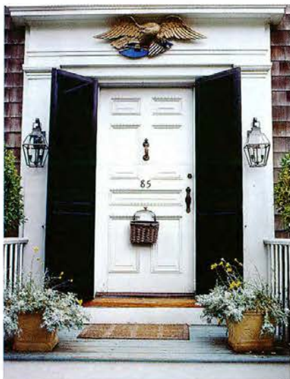
On Nantucket, a six-panel door is called Quaker-style and often dressed with shutters.
