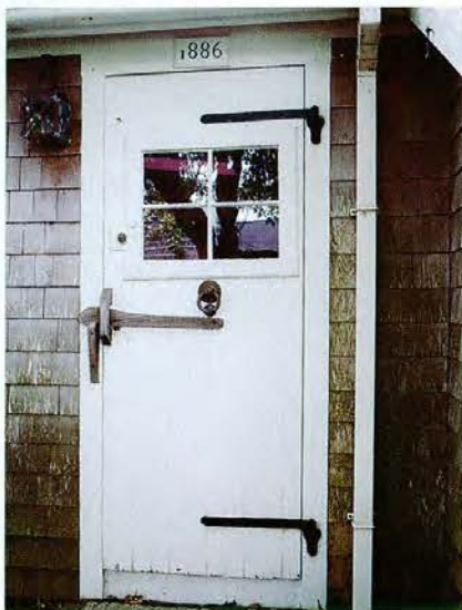
Strap hinges and bar latches were common elements of late-19th-century Nantucket style.
