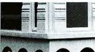
...sanded, nailed, stained or painted.
