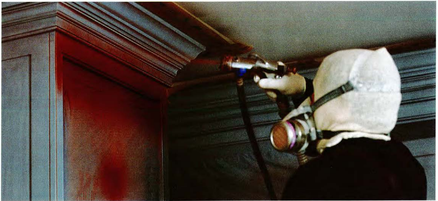
With skin, lungs and ceiling protected, Dee spray-paints crown moldings with his HVLP gun. For fine work, he restricts paint flow. “You can just about turn the gun into an airbrush,” he says, referring to an artist’s tool that paints with pinpoint control.
