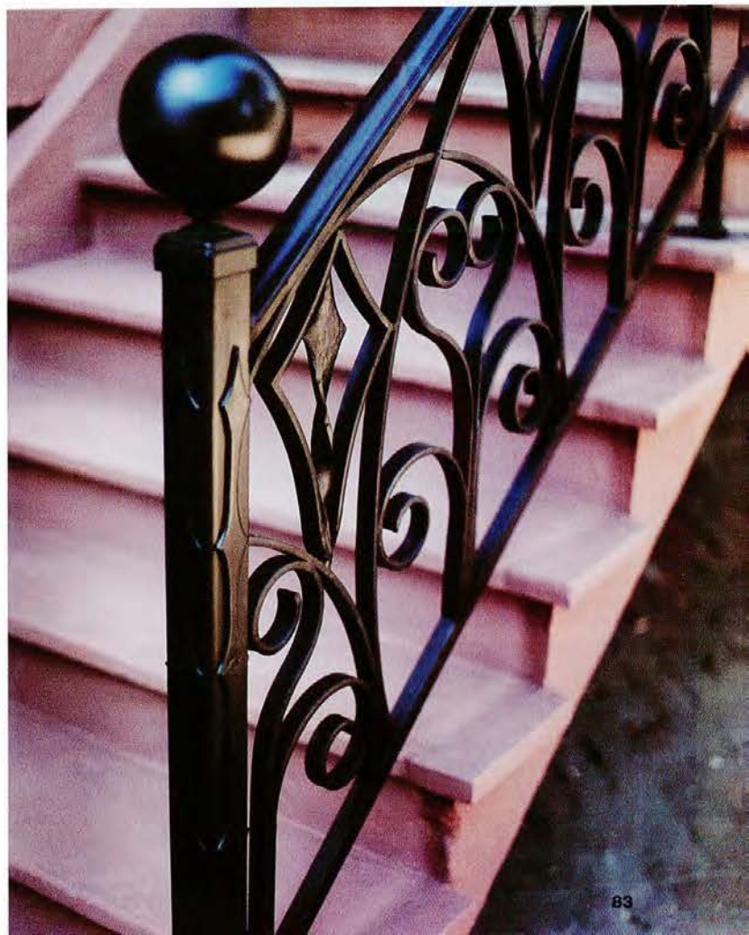
Smith hammers a scroll, above, until it's tight against a jig. Wrought iron railings often include scrolls because they keep children from falling through and they're easily formed. The same scroll in place at the Fleming house, below, where it echoes the home's original ironwork.
