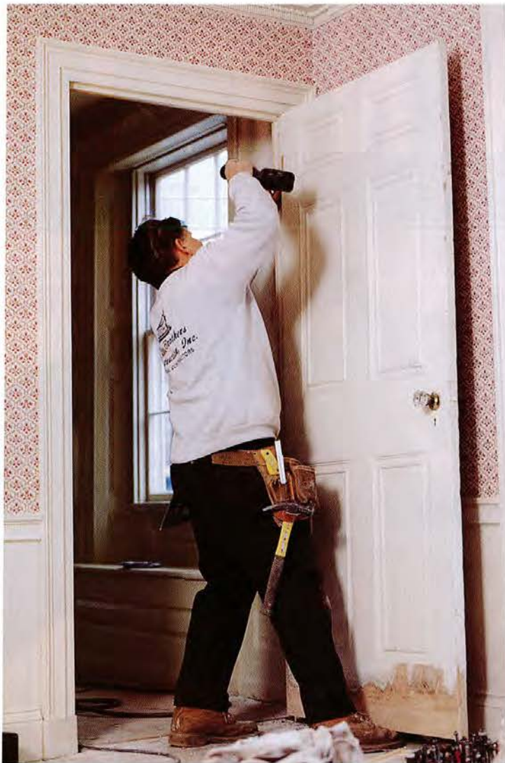
Work boots come in handy on this job. Balancing the door on his foot, Silva drives the first screw into the top hinge; another screw in the bottom hinge will suffice while he makes any fine adjustments. Drilling pilot holes into the mortises is an essential step.
