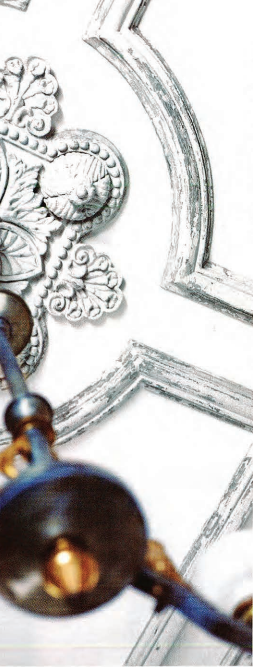
Coffered panel moldings at 2 East Taylor Street (1880) set off a richly detailed medallion with palmetto leaves, pearls and rosettes. This style resembles the handiwork of the Summerlin family, Savannah plasterers whose craftsmanship can also be seen in the city's cathedral.
