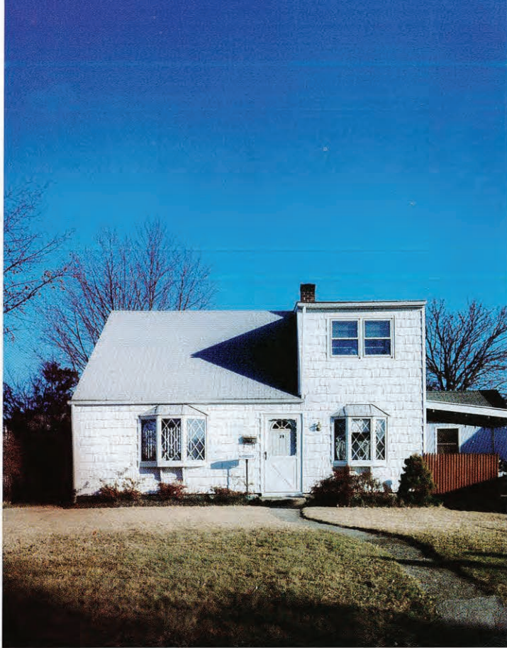
This Cape, now adorned with two diamond-pane bay windows, got its side dormer in 1978 and its shed extension in 1985.
