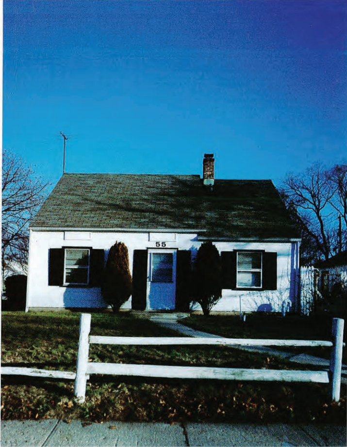
An almost original Type 2 Cape has a stepped-down roof and faux windows (now painted over) above a real window and the door.
