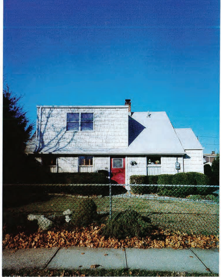
This house grew with the addition of a dormer in 1970 and a 4-by-12-foot side extension the following year.
