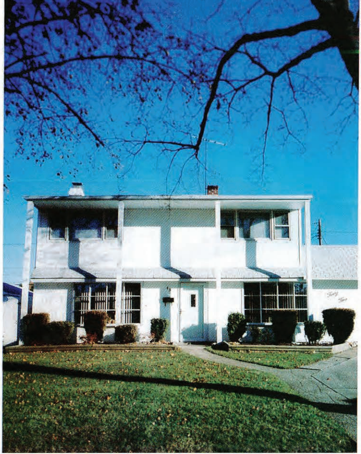
Beginning in 1970, this Cape evolved a style all its own. Changes include a full second floor, two-story pillars and an attached garage.
