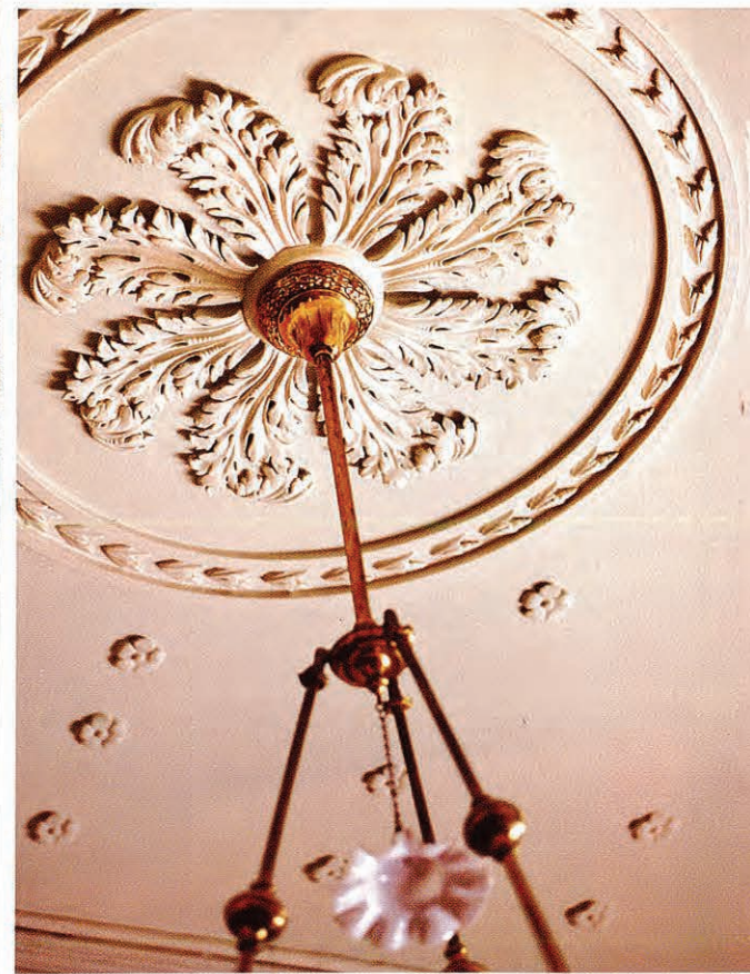
This medallion's turned acanthus leaves and enriched surround show off the Regency styling in vogue when the Wayne-Gordon House (142 Bull Street) was built in 1818. Note the rosettes arrayed across the ceiling.
