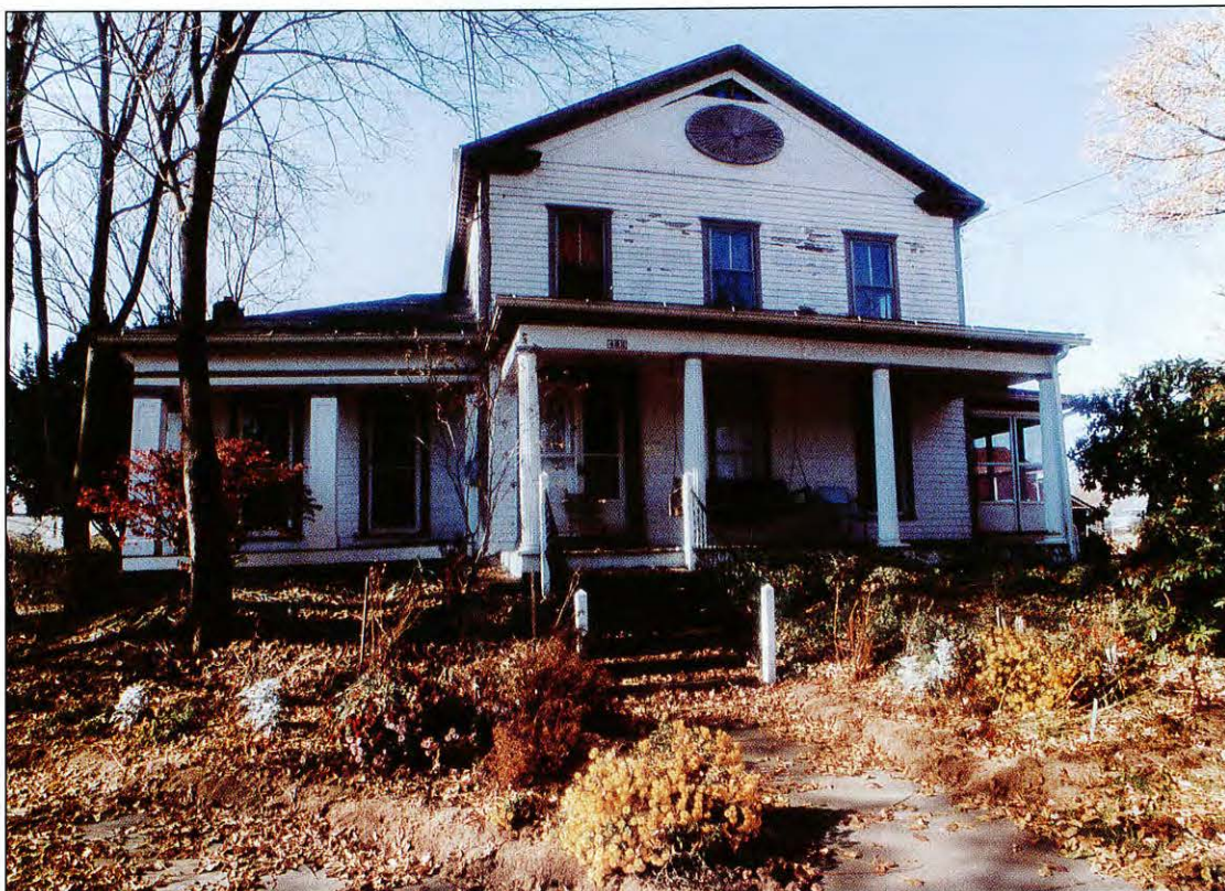
The house retains many Greek Revival details, including modillions on the eaves and a rosette molding.
