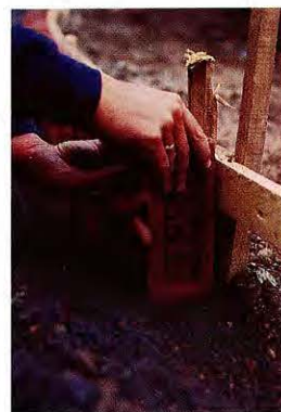
Brick work, p. 66
