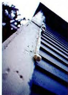
Foam that has expanded all the way to the outside is proof positive that it can seal otherwise inaccessible air leaks.
