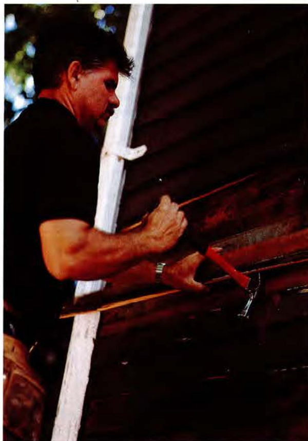
It took some getting used to, but now Tom Silva is crazy about this Yamaguchi with a long bent neck and extended handle. "It has extraordinary balance," he says, "and the long handle lets you get some beef into it for driving nails."
