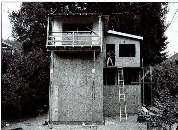
Raised 14 feet, 6 inches
