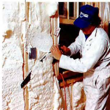
ABOVE: Open wall and roof framing is quickly filled in one or two passes. There's no need for roof vents because water vapor can't pass through the foam. LEFT: Minutes after the foam is applied, John Lojek trims off the excess with a handsaw. Trimmings don't go to waste: They're chopped up and used as loose-fill insulation in attic floors.
