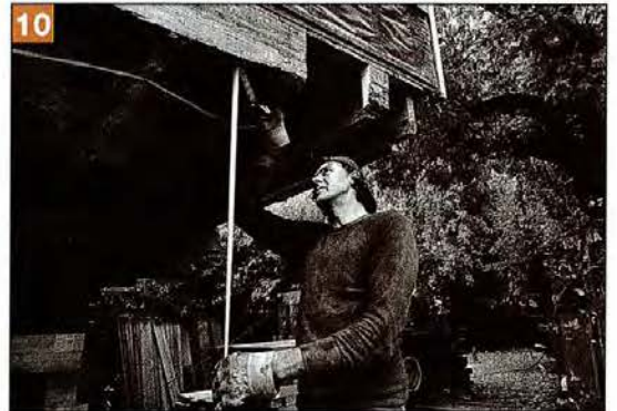
The actual lift takes only 5 minutes per foot. But resetting the jacks and stacking the cribbing requires more than an hour. The Coen house took two days to lift to its new height, rising 3 feet on the first day and 6 feet, 6 inches on the second.
