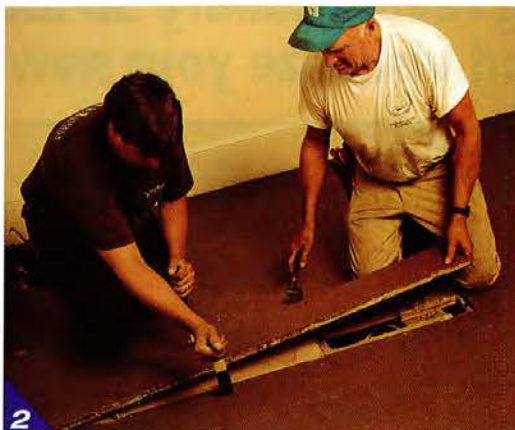
2 Bob Russell, an electrician familiar to This Old House viewers, and partner Joe Tremblay lift up the old pine floorboards, exposing the old-fashioned knob-and-tube wiring. They “fish” new electrical lines along this channel to the center of the room. (3) Pitard’s “pull” from the basement must go carefully so the cable doesn’t get pinched, knotted or stressed by too much pressure on the way up.
