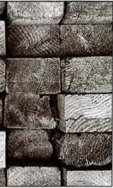
Cribbing timber is ready for stacking beneath the house.
