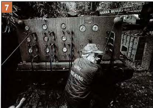
7 Archie Hanna of A.C. Hanna House Movers in Windsor, California, monitors pressure gauges to make sure the jacks, which carry different amounts of weight depending upon where they're located, are lifting at the same rate.
