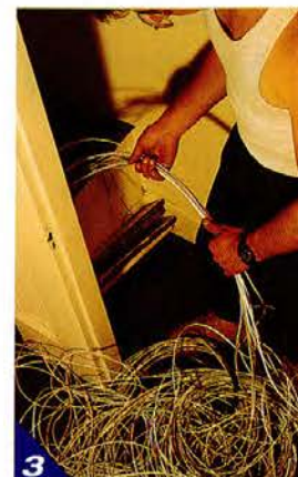
2 Bob Russell, an electrician familiar to This Old House viewers, and partner Joe Tremblay lift up the old pine floorboards, exposing the old-fashioned knob-and-tube wiring. They “fish” new electrical lines along this channel to the center of the room. (3) Pitard’s “pull” from the basement must go carefully so the cable doesn’t get pinched, knotted or stressed by too much pressure on the way up.
