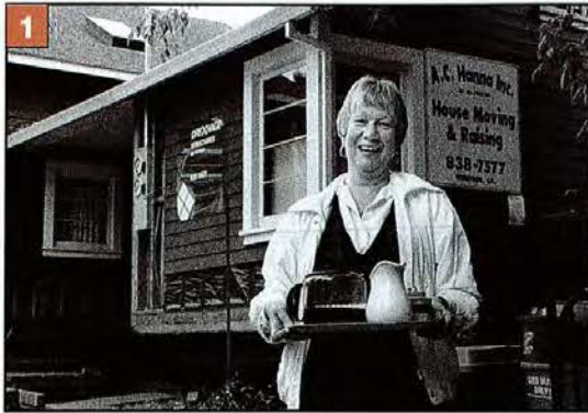
1 Barbara Coen's house sits on a steep embankment overlooking the Russian River. During the floods last winter, water covered the dining-room table. Raising the house 9 and a half feet will put it 1 foot above the 100-year flood level.
