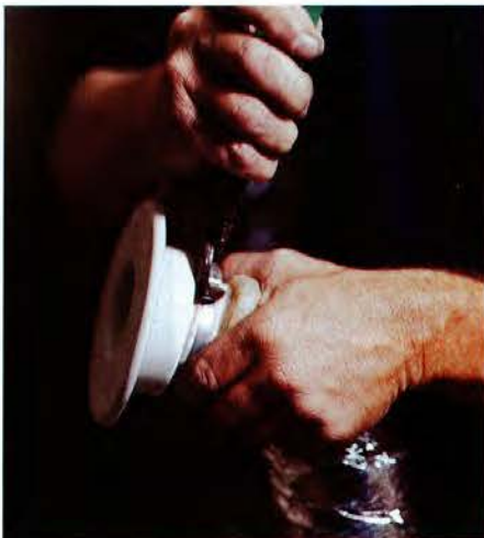
The outlet finish plate slips easily into the end of the duct. It is then clamped tightly to prevent possible air leaks.
