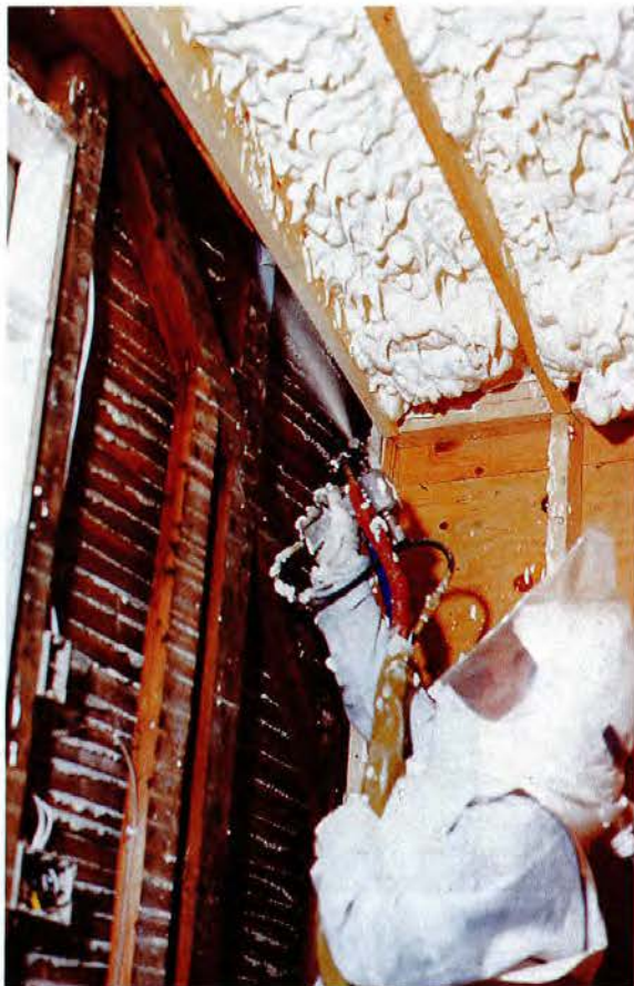
ABOVE: Open wall and roof framing is quickly filled in one or two passes. There's no need for roof vents because water vapor can't pass through the foam. LEFT: Minutes after the foam is applied, John Lojek trims off the excess with a handsaw. Trimmings don't go to waste: They're chopped up and used as loose-fill insulation in attic floors.
