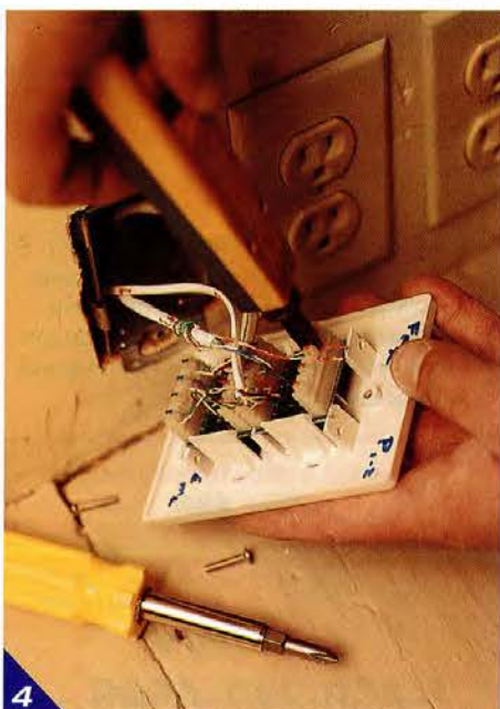
1 Only one ungrounded electrical outlet served the new home office, and there was no phone jack. The closet offered access to the heating duct, a handy channel Bob Pitard used for pulling up the cable from the basement.
