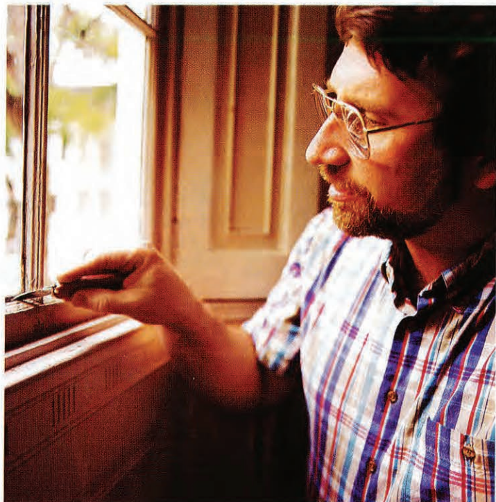
ABOVE: Anywhere water can collect, you're likely to find rot, says Norm, who found plenty around the trim on the bay window. BELOW: Although the house has no storm windows and ice must form easily on the inside in winter, Norm found almost no rot in the mullions and sash.
