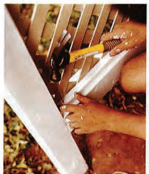
8 Nail post bases to blocks using masonry nails provided with post bases. Set lattice frame into bases and level, then attach with 4d common nails. Toe an 8d common nail through each rafter to secure. Prime frame and stops. Install outside stops using 8d finish nails. Install lattice and inside stops.
