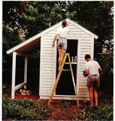
10 Trim fascia and rake. Install fascia using two 8d finish nails in each rafter and rake using 8d finish nails 16" on center. Prime trimmed ends. Install cornerboards and door trim with 8d finish nails. Install battens with sinkers 8" on center and ridge roll with 1" roofing nails 12" on center. Caulk batten covering ply joint.
