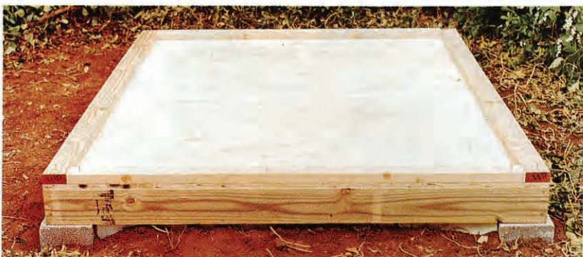
4 Dig trough around the inside of the frame and set flashing at least 4" deep. Backfill trough. Remove brace and lay back-primed ply flooring , making sure the joint lays on a joist. Using 8d sinkers, nail down the plywood at 8" on center. Rough tack 2x4 sole plates and mark stud locations 24" on center.
