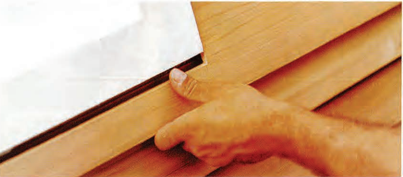
13 To fit a clapboard under the window , measure where the window hits the clap. First make vertical cuts with the circular saw, then score the horizontal cut with a utility knife and straightedge. Snap off the clapboard. Caulk claps where they meet window, door and cornerboards. Countersink all finish nails, putty in holes.
