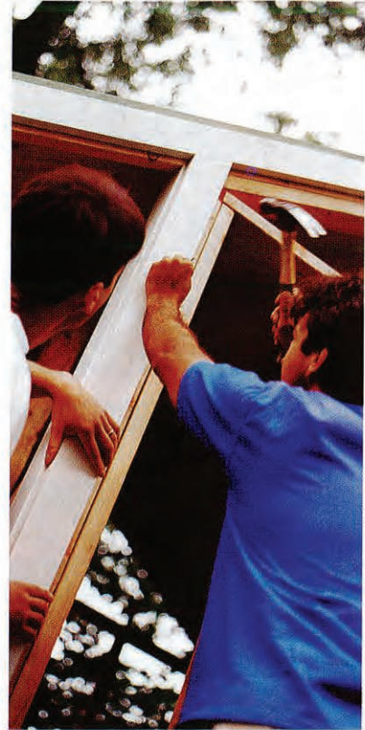
10 Trim fascia and rake. Install fascia using two 8d finish nails in each rafter and rake using 8d finish nails 16" on center. Prime trimmed ends. Install cornerboards and door trim with 8d finish nails. Install battens with sinkers 8" on center and ridge roll with 1" roofing nails 12" on center. Caulk batten covering ply joint.
