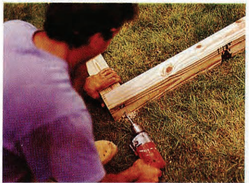
7 Dig the holes for the blocks that will support the lattice posts, sinking blocks below grade (ground level). Measure and cut each 4x4 to fit under a rafter. Double-check the squaring as you bolt together the lattice frame . Pre-drill bolt holes using a 1/4" drill bit. Install lag bolts and then tighten with a wrench.
