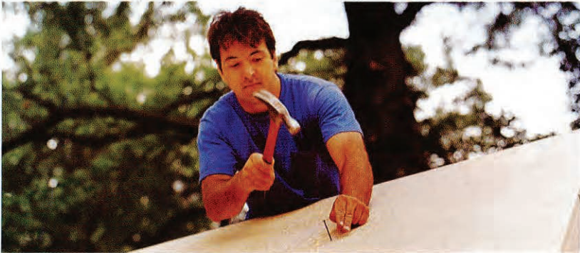
9 Nail hurricane anchors to rafters with 4d commons. Install roof sheathing , placing one sheet of ply horizontally on the short side, two sheets vertically on the long side. Make sure sheets abut on the center rafter. Use chalk line to mark rafter locations, then nail down plywood with 8d sinkers 8" on center.
