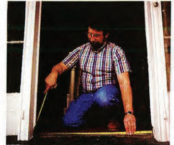
ABOVE: Norm snugs blade into doorway. BELOW: Length of flat tape plus estimate of gap equals total: 34 1/4 inches.
