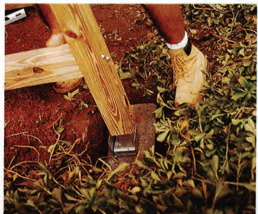
4 Dig trough around the inside of the frame and set flashing at least 4" deep. Backfill trough. Remove brace and lay back-primed ply flooring , making sure the joint lays on a joist. Using 8d sinkers, nail down the plywood at 8" on center. Rough tack 2x4 sole plates and mark stud locations 24" on center.
