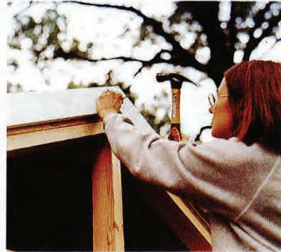
10 Trim fascia and rake. Install fascia using two 8d finish nails in each rafter and rake using 8d finish nails 16" on center. Prime trimmed ends. Install cornerboards and door trim with 8d finish nails. Install battens with sinkers 8" on center and ridge roll with 1" roofing nails 12" on center. Caulk batten covering ply joint.
