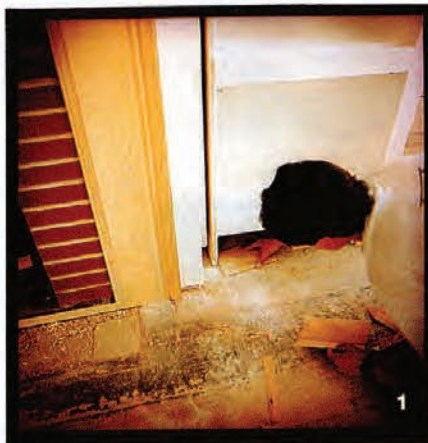
(1) After the boxes are completed, installation begins; about one-third of the work is still ahead. First, Encalada sets one bottom box in place. The case tilts toward the fireplace, so he pushes short pieces of shingles under the base on that side. (Shingles make good shims because they're tapered.) (2) When the cabinet appears level, he checks by laying a 2-foot level across the top. After several adjustments, he's satisfied
