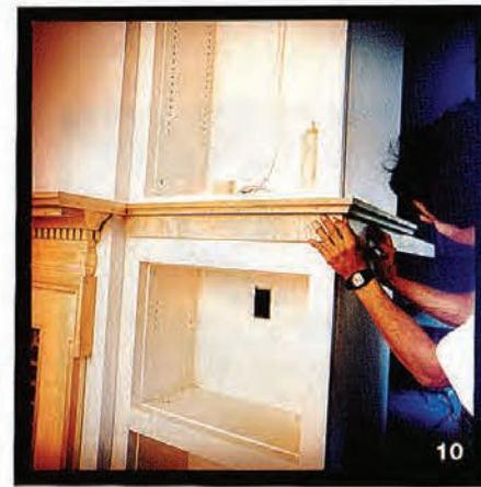
(9) Ribbons of molding tie this bookcase to the room. Trim carpenter Robert Caruso applies the crown molding, often tricky because corners are rarely perfectly square. He cuts two short pieces to test the angle of the miter cut, so he won't waste time coping the other end of a piece that doesn't fit. (10) The middle molding in this design is built up from several pieces and continues around a corner into the next room.
