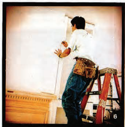
(5) Once the bottom is secure, the top cabinet is lifted into place. Leveling isn't necessary, because the base is level. Encalada simply screws the top box to the walls. (6) He holds the side frame piece in place (the part that wasn't glued on back at the shop) so it can be fitted to the wall. He uses a compass, adjusted to the gap between the wall and the wood, to transcribe irregularities in the wall to the edge of the frame piece.
