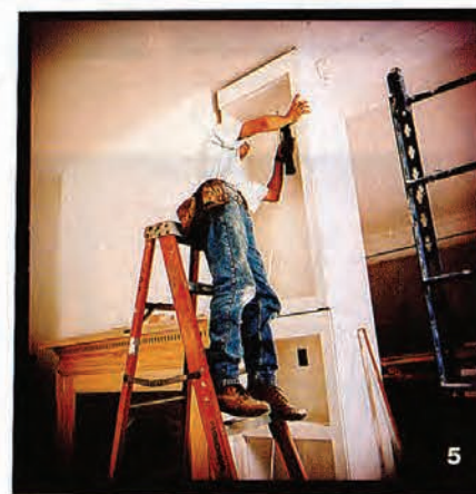
(5) Once the bottom is secure, the top cabinet is lifted into place. Leveling isn't necessary, because the base is level. Encalada simply screws the top box to the walls. (6) He holds the side frame piece in place (the part that wasn't glued on back at the shop) so it can be fitted to the wall. He uses a compass, adjusted to the gap between the wall and the wood, to transcribe irregularities in the wall to the edge of the frame piece.
