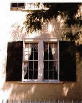
Rea House, 1835 20 Chestnut Street
