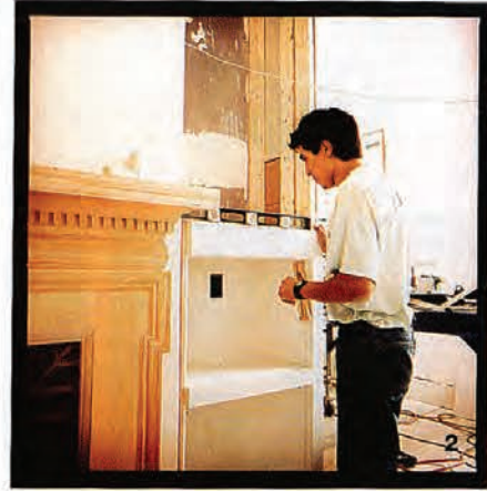
(1) After the boxes are completed, installation begins; about one-third of the work is still ahead. First, Encalada sets one bottom box in place. The case tilts toward the fireplace, so he pushes short pieces of shingles under the base on that side. (Shingles make good shims because they're tapered.) (2) When the cabinet appears level, he checks by laying a 2-foot level across the top. After several adjustments, he's satisfied
