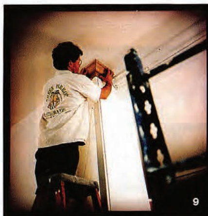
(9) Ribbons of molding tie this bookcase to the room. Trim carpenter Robert Caruso applies the crown molding, often tricky because corners are rarely perfectly square. He cuts two short pieces to test the angle of the miter cut, so he won't waste time coping the other end of a piece that doesn't fit. (10) The middle molding in this design is built up from several pieces and continues around a corner into the next room.
