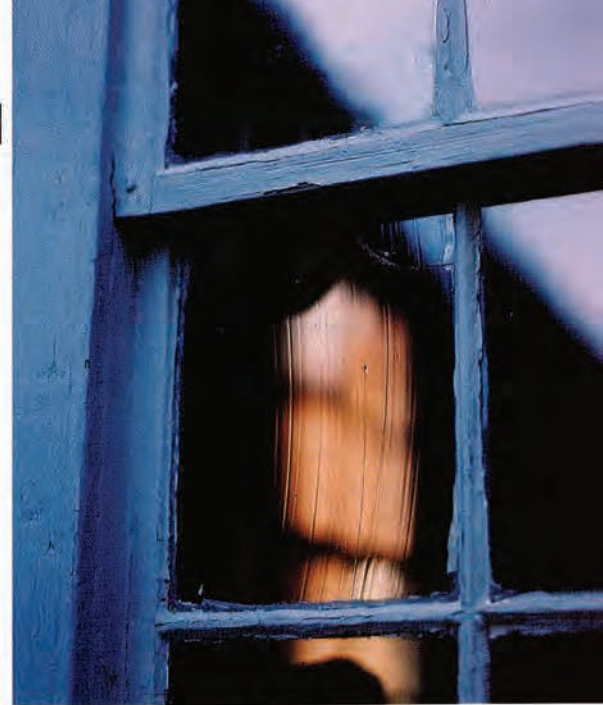
The curved striations in this old pane are the telltale signature of crown glass.
