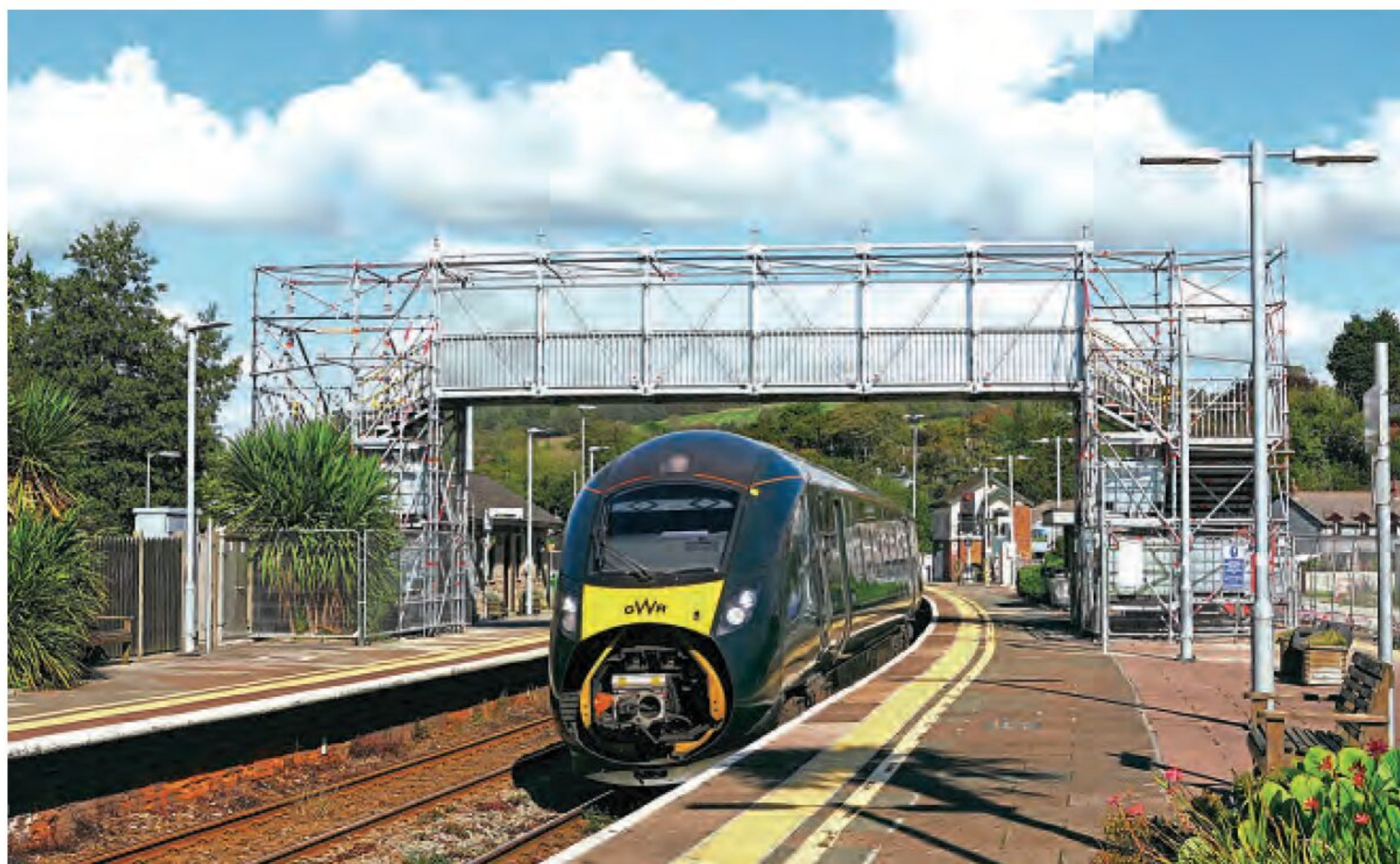
A temporary footbridge has been installed at Lostwithiel (Cornwall) to allow passengers to cross between the platforms without using the level crossing at the eastern end of the station, which is now closed more often following an increase in the train service frequency. The basic structure, which includes scaffolding and alloy panels, will be replaced in the long-term with a permanent structure. No. 800311 passes beneath the footbridge on October 3 with the 10.03 Paddington to Penzance. JOHN VAUGHAN
