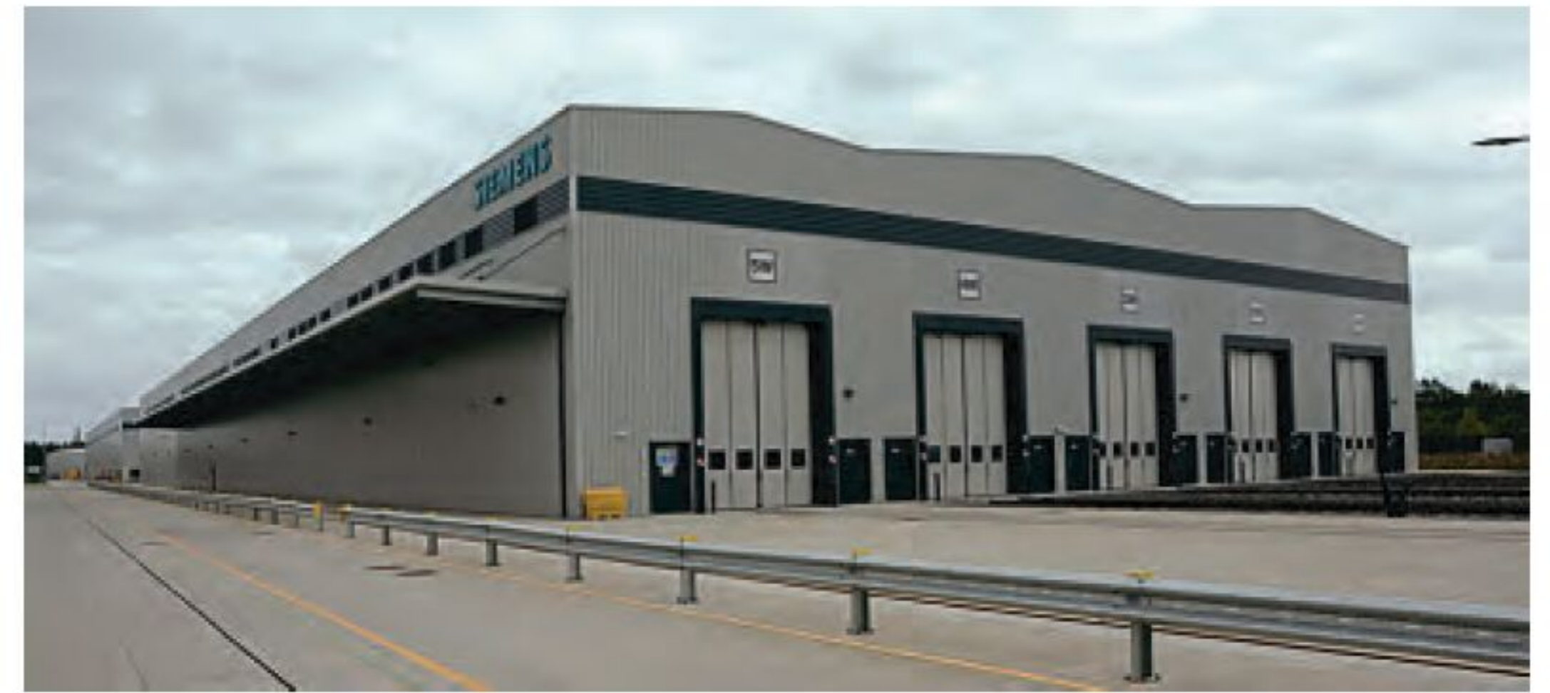
One of the huge new buildings that make up the Goole Train Manufacturing Facility.
