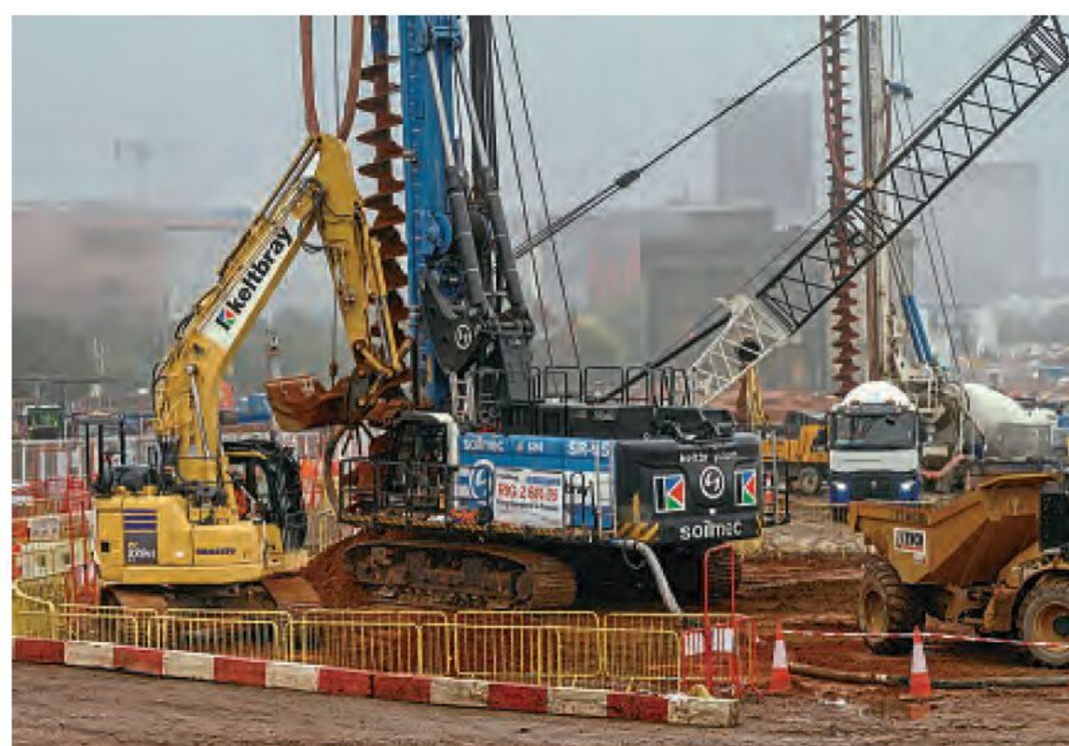
With a backdrop including the Grade I-listed entrance building to the long-demolished London & Birmingham Railway Curzon Street station, work is underway to create the foundations of the adjacent station of the same name that will be used by HS2 trains serving Birmingham. HS2
