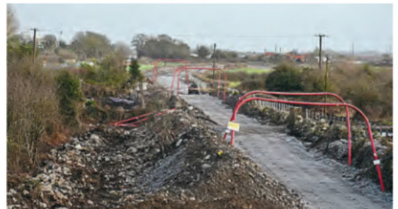
Tracklaying is expected to start on the Foynes reinstatement project this spring (quarter two of 2024). Work on laying the final ballast base began just before Christmas when a trial layer was installed at Morgons South, near MP 23½ between Askeaton and Foynes. The freshly laid ballast can be seen on December 21, looking towards Limerick with main contractor Sisk's compound in the distance. HASSARD STACPOOLE
