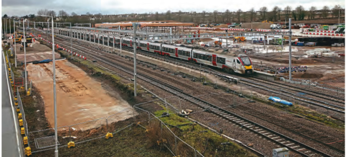
Greater Anglia EMU No. 745005 on the new Down Main alignment through the Beaulieu Park station site with 1P34, the 14.00 London Liverpool Street-Norwich on January 2. The disconnected and part lifted former main lines are in the foreground. DRAIN C SCOTCHMAN
