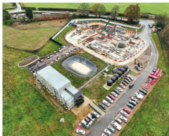
The work site at the 42 metre (138 feet) deep shaft at Chesham Road near Great Missenden, one of five which will provide emergency access to the Chiltern tunnel. The tunnel boring operation below had reached this point by mid-December. HS2
