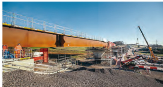
The bridge deck push at Wendover Dean Viaduct is seen in its initial stages last month. HS2
