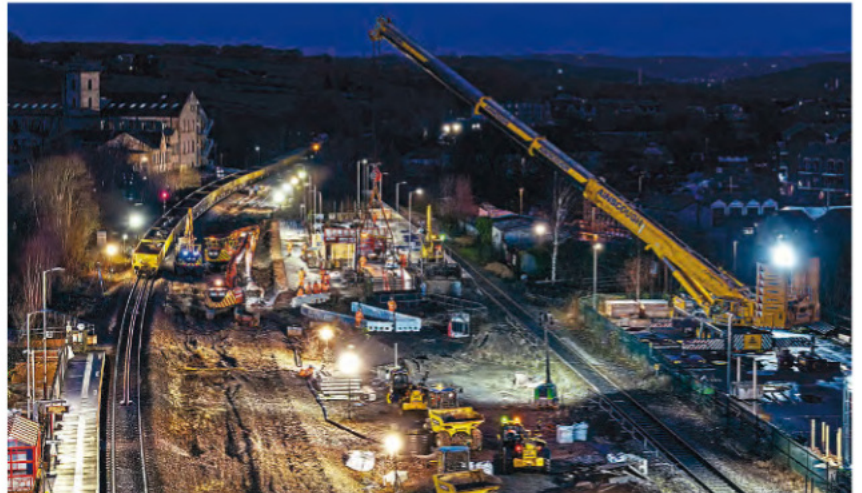
TransPennine Route Upgrade work taking place at Mirfield station during the Christmas and New Year period. NETWORK RAIL
