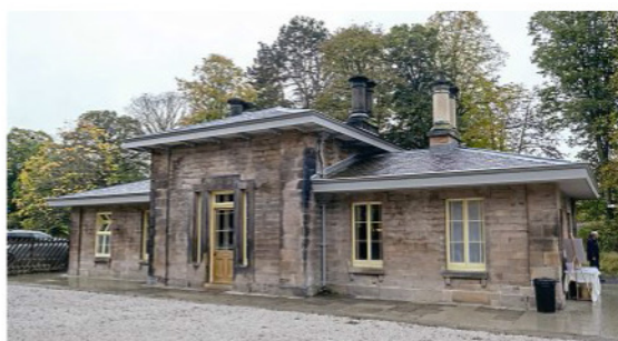
A remarkable and worthy transformation of Wingfield station showing the completed restoration work as seen on October 28. Trains regularly pass by the station at speed and can be safely viewed from behind fencing. A footpath runs through the station site so makes the building accessible. CHRIS MILNER
