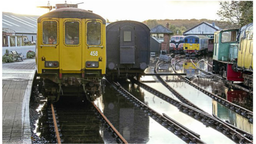
As 5ft of flood water subsided, the DCDR could begin to assess the substantial damage that had been caused.
