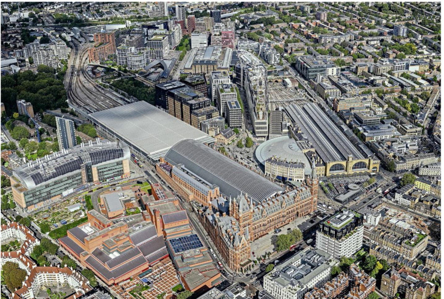
Just east of Euston are the Midland Main Line and East Coast Main Line termini at St Pancras and King's Cross respectively. St Pancras is on the left of this northwards view, showing the ornate George Gilbert Scott-designed brick building, its original arched trainshed and the flat-roof extension added when the station became the home of Eurostar international services in 2007. To the right is the more compact, Lewis Cubitt-designed King's Cross, and between the two stations are the recently built buildings as part of the regeneration of the area.
