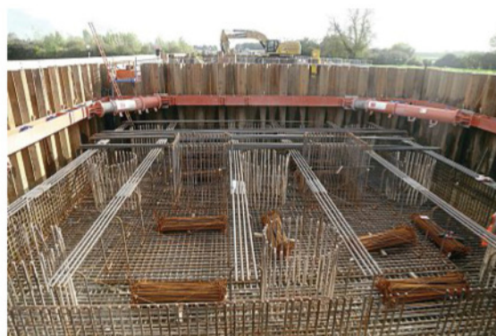
One of the viaduct's pier foundations under construction.
