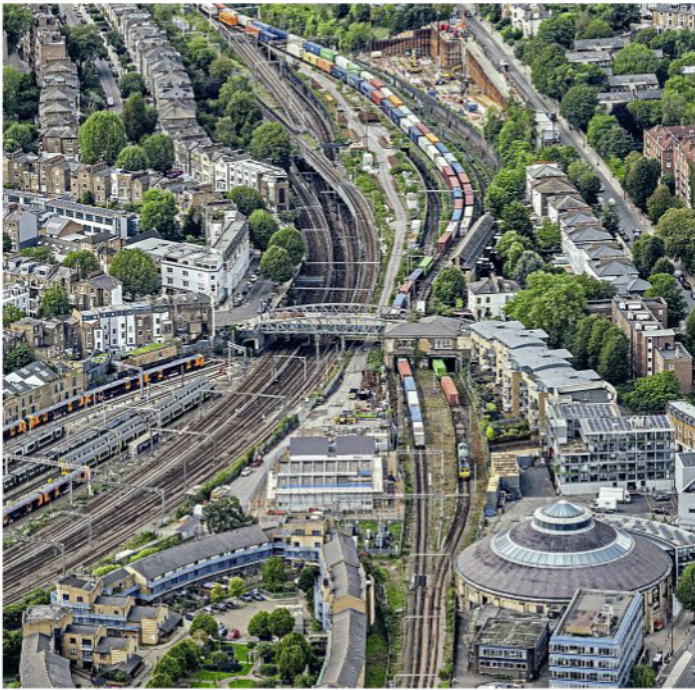
North-east of Marylebone, across Regent's Park, is the former station at Primrose Hill (closed 1992) – the overgrown island platform on the connection between the West Coast Main Line and North London Line can be seen in the centre of this shot between the two intermodal trains. Adjacent to the closed station is the Camden Roundhouse, a locomotive shed from 1837 to 1966 but now a music and arts centre, while on the left are a number of EMUs stabled in Camden Carriage Sidings.
