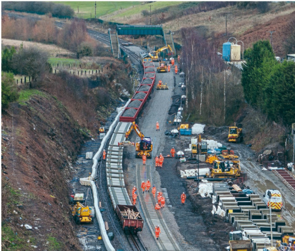
The Government has committed to large rail projects such as the TransPennine Route Upgrade – which included this work over Christmas towards resiting the station at Morley to allow electrification and raised linespeeds. NETWORK RAIL
