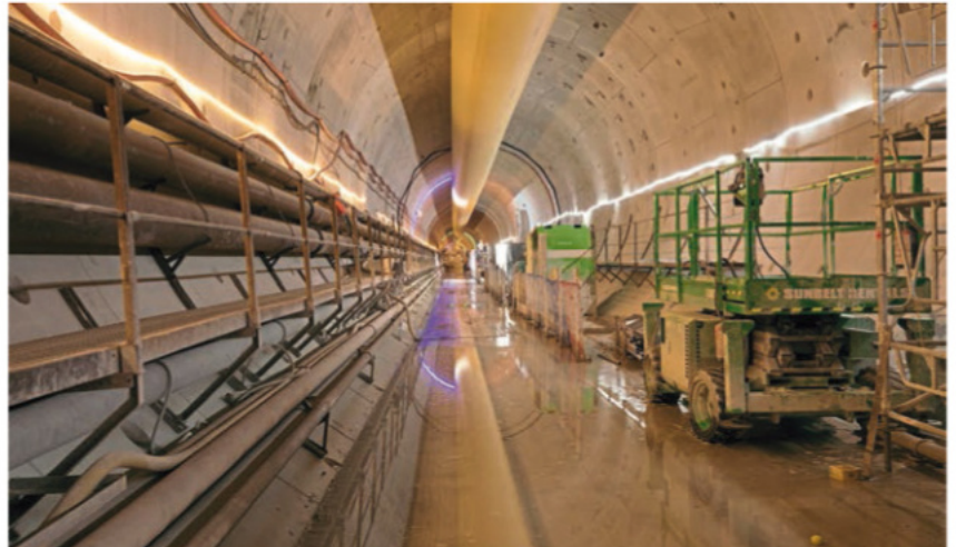
A lined section of the tunnel with some of the equipment being used to complete its construction. HS2
