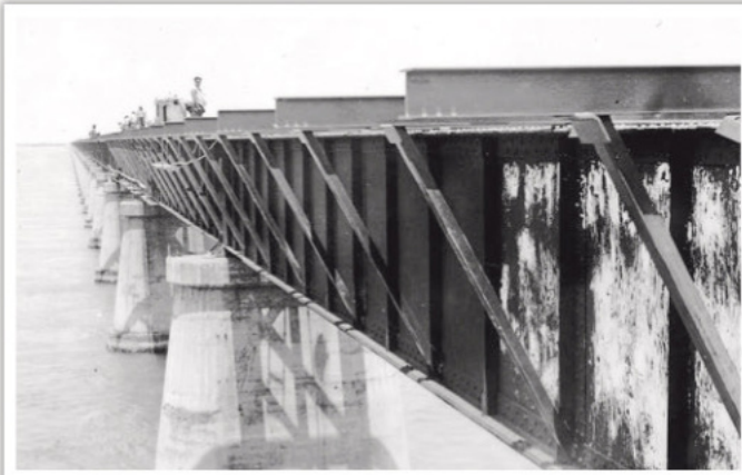
After closure, much of the railway was converted into a road, this view showing supports being added to the Seven Mile Bridge for a two-lane highway. FLORIDA KEYS HISTORY CENTER (CC BY 2.0)
