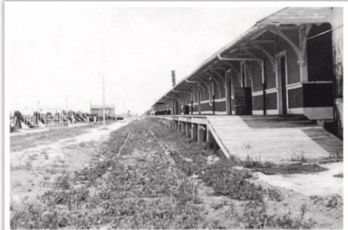
The abandoned station at Key West after most of the track had been lifted. FLORIDA KEYS HISTORY CENTER (CC BY 2.0)
