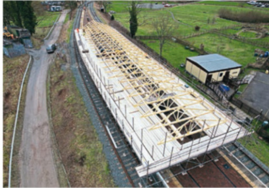
Corwen station canopy seen from above. Installation of roof panels was well underway by mid-February. The car park is on the right while the signalbox is just visible at the top of the image. RICHARD WALLIKER/LRT
