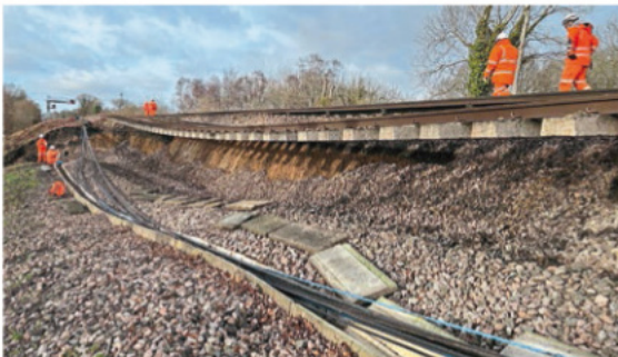
Above: A close-up of the landslip on the embankment under the down slow line near Hook. NETWORK RAIL
