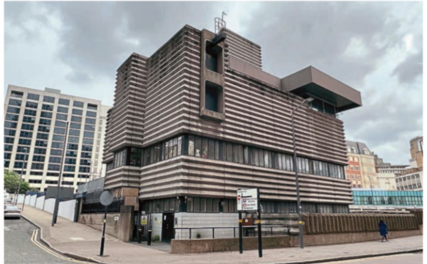
Birmingham New Street's Grade II Listed 1960s signalbox closed on December 24. NETWORK RAIL
