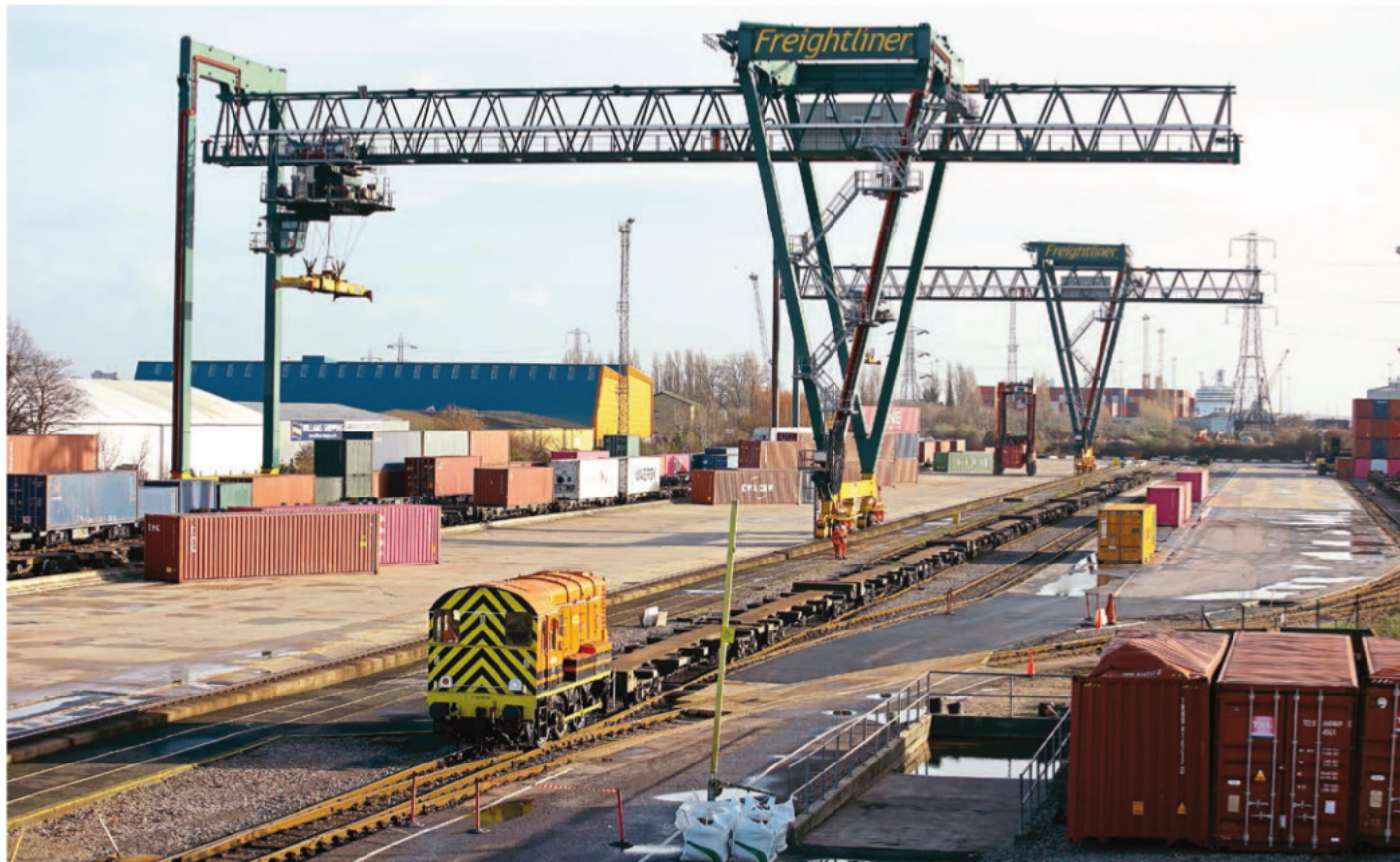
After a long spell working at Ipswich, Class 08 shunter No. 08785 has returned to Southampton Maritime Container Terminal, where it is seen at work on December 29. It is dwarfed by the two Liebherr gantry cranes which load the boxes deposited on the pad areas by a fleet of straddle carriers that shuttle between the MCT and various deep-water berths. STEVE STUBBS
