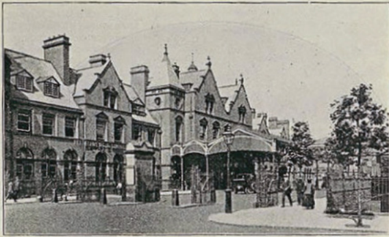
HEADQUARTERS OF THE LONDON AND NORTH EASTERN RAILWAY, MARYLEBONE STATION, LATE GREAT CENTRAL RAILWAY.
