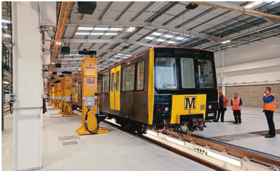
METRO MOVES IN: Staff began to move into the Tyne & Wear Metro's new £70 million depot at Gosforth in Newcastle in late November. Metrocar No. 4062 is pictured having entered the maintenance shed for the first time. The facilities, created in readiness for the system's new fleet of 46 Stadler trains, also include a separate wheel lathe building and train washing plant. They have been built alongside the old depot, which is being demolished. NEXUS
