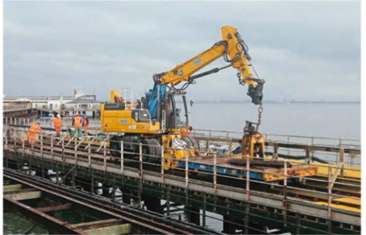
A road-rail vehicle on the railway pier on November 14. Network Rail is using the closure of the pier to also upgrade the remaining single track running line.
