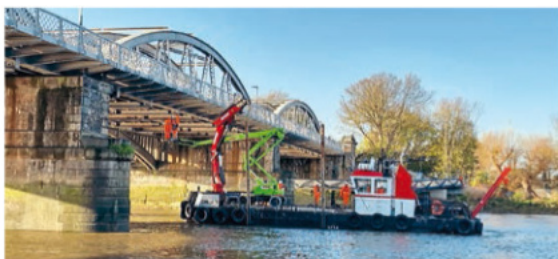
Network Rail engineers replaced a number of the securing pins in the girders of Barnes Bridge using a combination of scaffolding, abseiling and a hydraulic 'cherry picker' lift on a boat on the River Thames. NETWORK RAIL
