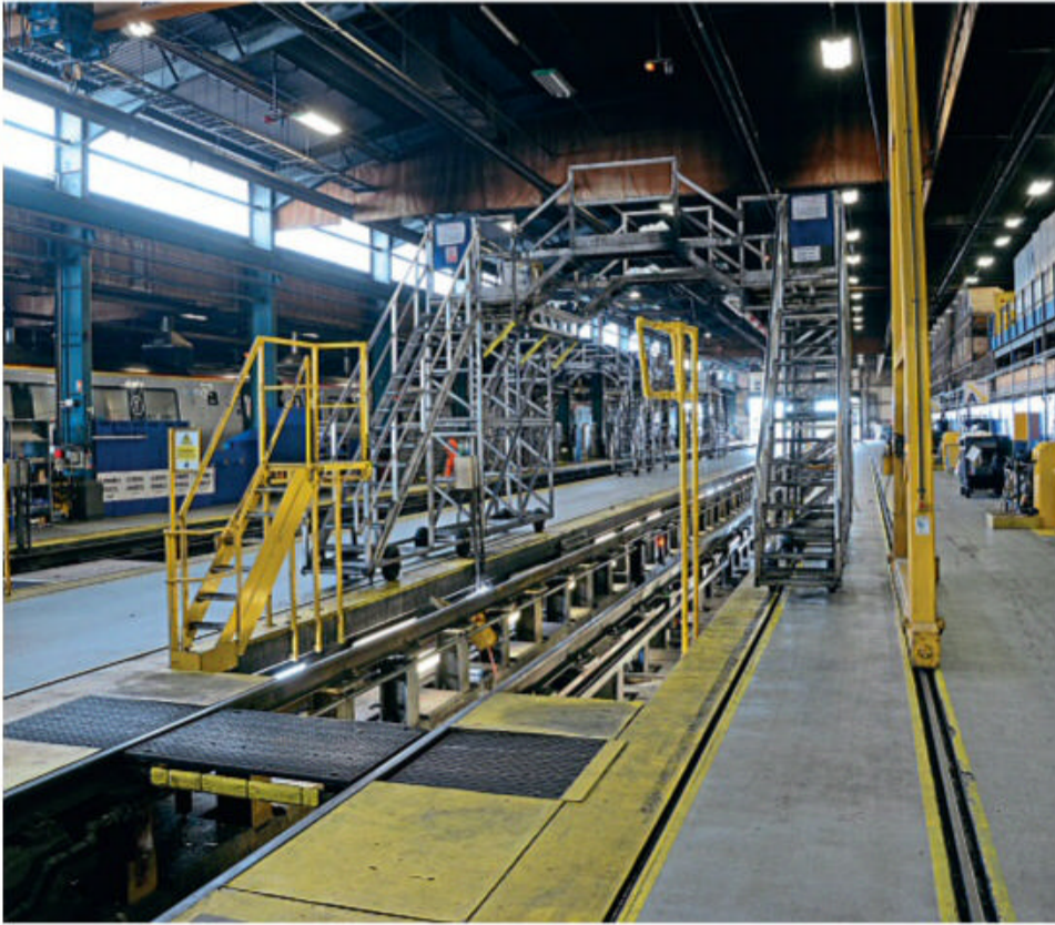
Above: The two-road middle maintenance shed, where the ladders allow access to the roof-mounted equipment such as the heating, ventilation and air-conditioning (HVAC) units.
