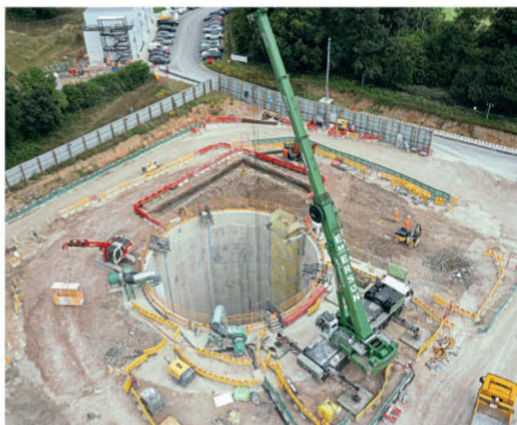
The shaft at Chalfont St Peter pictured in July. HS2
