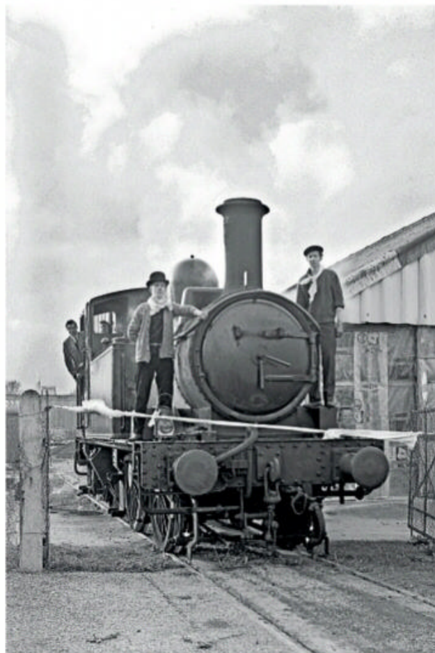
The first (unplanned) steaming of No. 1466 at Totnes in April 1964. GWS
