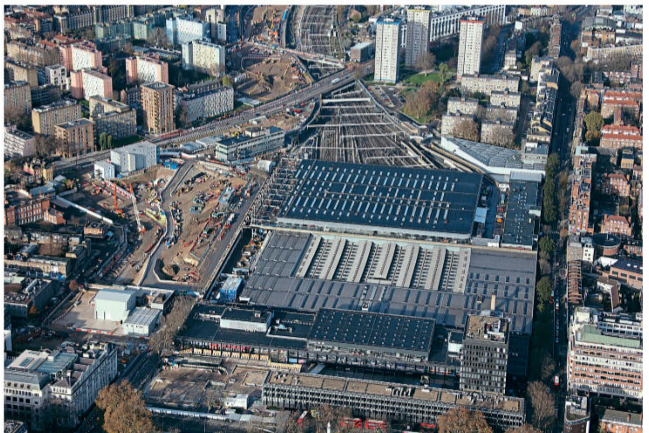
Looking north over Euston on November 22, 2020 showing the works to the left (west) side for HS2.
