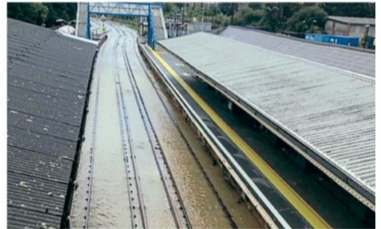
Flooding at Ryde St John's Road station on August 2. SWR
