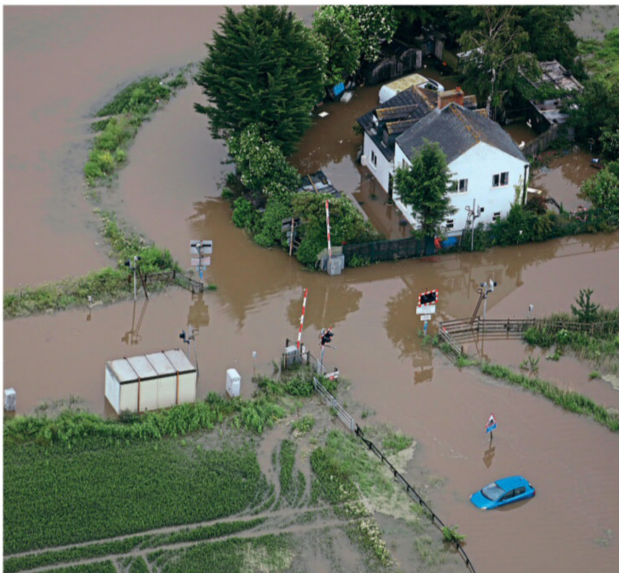
It does not need a high-resolution camera to spot the problem here – but the helicopter gives a view of the inaccessible level crossing at Brewster Lane, near Boston, on June 14, 2016.
