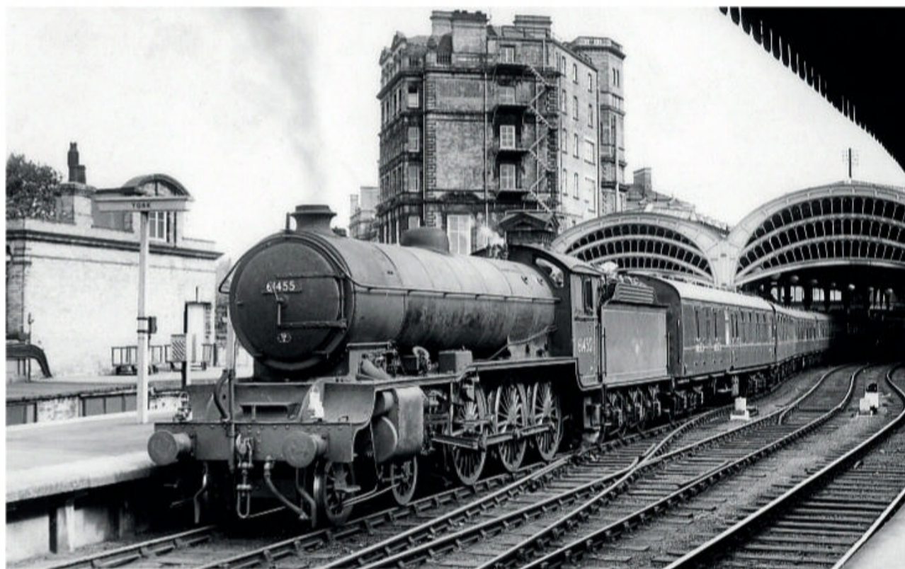
In the bays at the north end of York station, 'B16/2' No. 61455 heads the 5.16pm train to Hull via Market Weighton on June 20, 1961. S CREER
