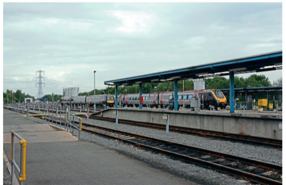
The north end of the cleaning and stabling sidings looking towards the fuelling area and wash plant. Three-car CrossCountry Class 170 No. 170638 awaits its next duties alongside XC 'Voyager' No. 221125.
