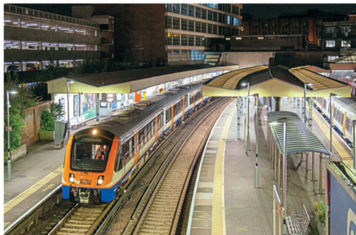
New London Overground unit No. 710378 was on test with ROG in the early hours of July 31, the unit pictured at Richmond ready to work a circular trip via Clapham Junction. FRASER HAY
