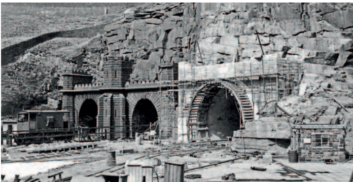
Below: A view at Woodhead on August 2, 1953, of the new tunnel being built alongside the old tunnels. WALTER DENDY/CC BY-SA 2.0
