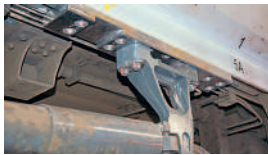
The new spreader plate fixed into the 'T' section on the bodyside.
