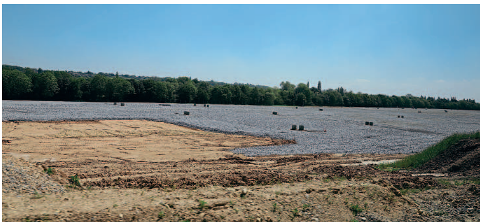
Extracted tunnel material storage will be stored on site until used for landscaping the completed project.
