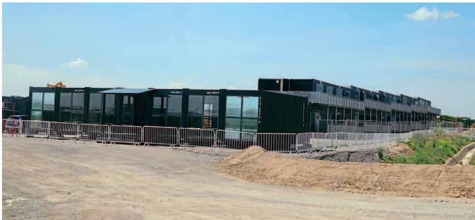
This pop-up hotel has been built on site for the tunnelling team.
