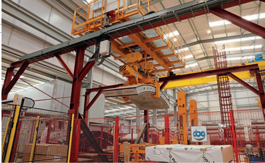
A concrete segment produced in the on-site production line.
