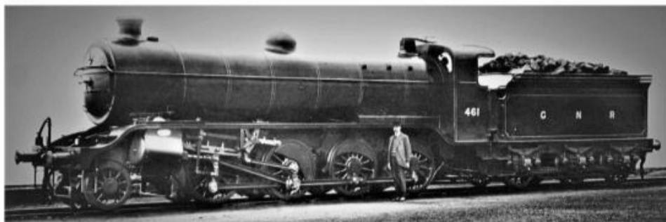
Above: Gresley wanted to take his '02' 2-8-0 design a step further and explore the use of three cylinders equipped with a two-in-one conjugated valve gear. This concept became a trademark part of his designs for the next 20 years. Here he poses before his first locomotive, No. 461, to be so fitted. Many more 2-8-0s would follow, but it was his Pacifics that would grab headlines and make his name.
