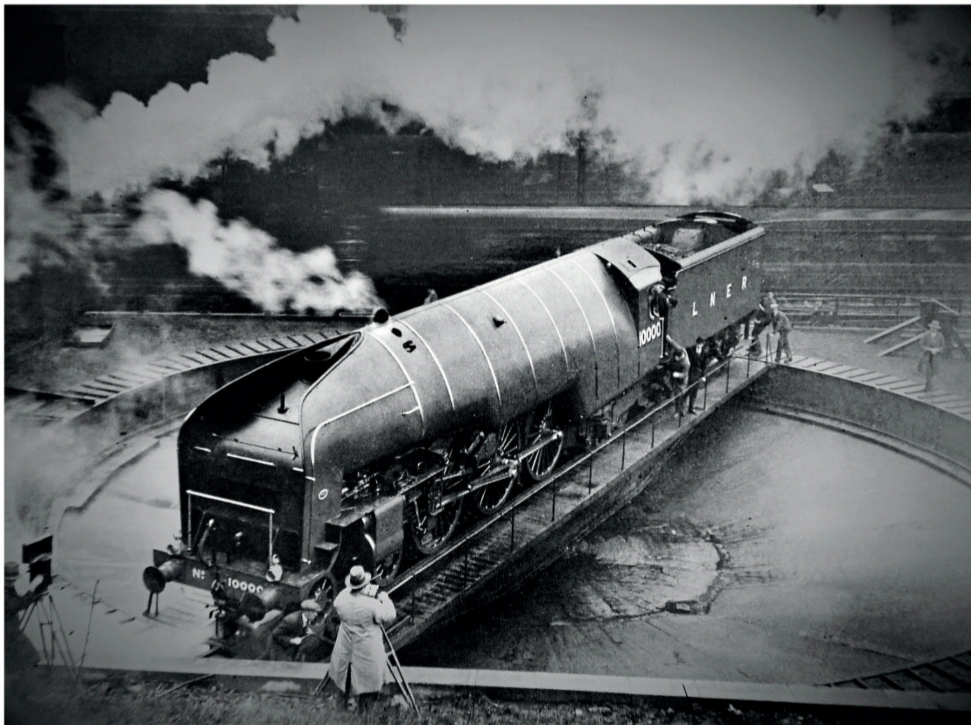
Below: 'W1' 4-6-4 No. 10000 – Gresley's attempt to take steam locomotion a giant step forward. With its four cylinders, high pressure water tubed boiler and a degree of streamlining, it certainly attracted attention. Here a newsreel cameraman films this unique locomotive on the turntable at King's Cross. AUTHOR
