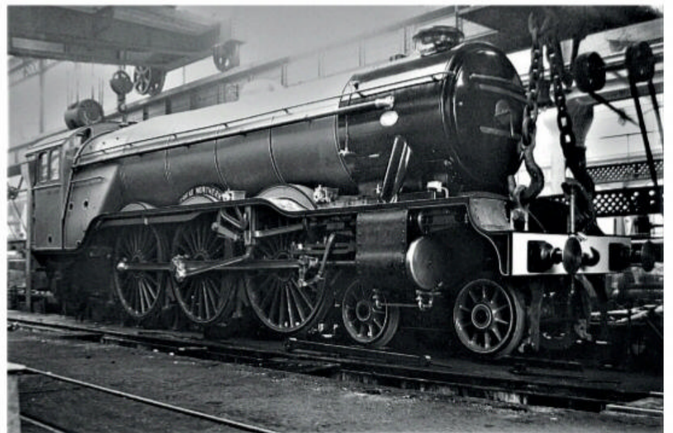
Above: Gresley wanted to take his '02' 2-8-0 design a step further and explore the use of three cylinders equipped with a two-in-one conjugated valve gear. This concept became a trademark part of his designs for the next 20 years. Here he poses before his first locomotive, No. 461, to be so fitted. Many more 2-8-0s would follow, but it was his Pacifics that would grab headlines and make his name.
