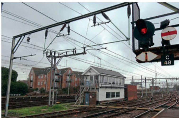
The 57-lever GER Type 7 Clacton-on-Sea signal box, dating from 1891. It is seen here on February 21, 2017. RICHARD HORNER
