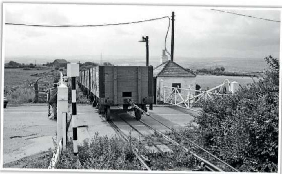
Waggons pictured on the Mount Level Crossing at Eighton Banks on August 15, 1993. The consist is on the Blackham's Fell West Incline, also known as the 'Short Bank', which is 750 yards in length. Blackham's Hill hauler is further up the hill behind the camera, with the Blackfell hauler building visible on the left of the picture, above the crossing gate. TREVOR ERMEL
