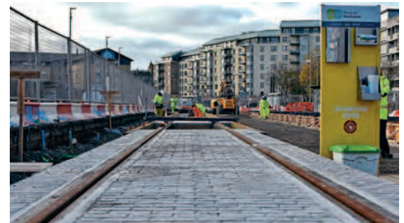
The first tracks are laid at the future Ocean Terminal stop in Leith. EDINBURGH COUNCIL
