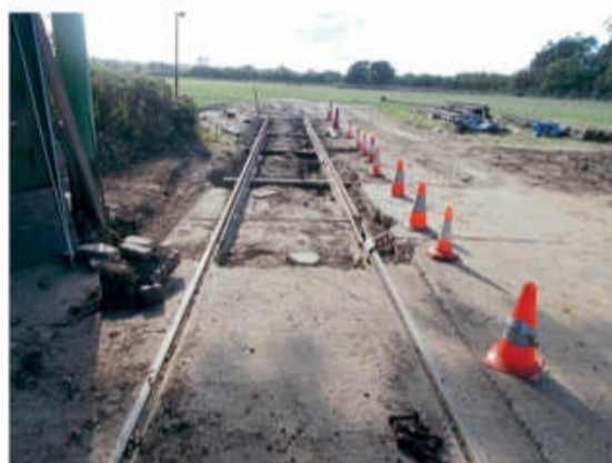
The first rails to be installed on the western extension of the East Anglia Transport Museum tramway looking towards the site of the proposed tram depot. TIM MAJOR
