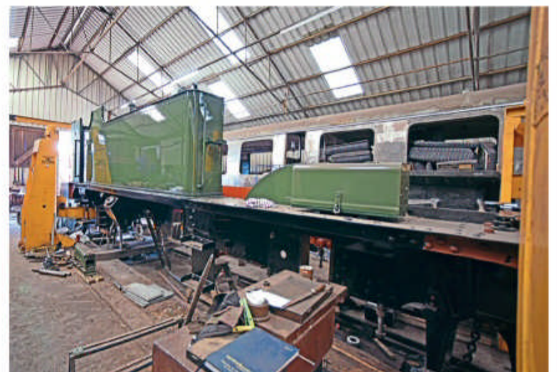
Work is progressing on the overhaul of the Great Western Society's '14XX' No. 1466 at Western Steam Engineering, last month seeing the fitting of one of the newly fabricated side tanks. The originals were very badly corroded. PHILIP MORRELL/GWS
