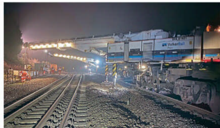
Two Volker Rail Kirow cranes were drafted in at short notice to assist with the emergency replacement of a switch at Aynho Junction, near Banbury, on November 7. NETWORK RAIL
