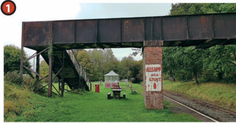
1. Looking east at the Bala Lake Railway's current terminus at Pen-y-Bont. The extension will leave the main line behind the camera, then pass beneath the left-hand span of the footbridge and curve sharply northwards along the fence line in the distance.
