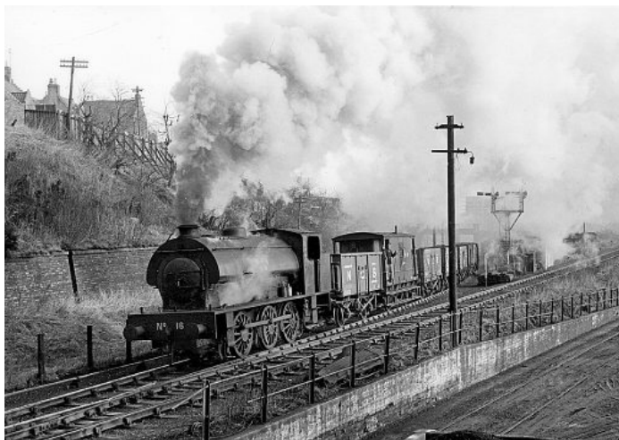
INDUSTRIAL STEAM FOCUS: Steam may have ceased on BR, but there was attention on industrial locations. Wemyss Private Railway Bagnall 'Austerity' 0-6-0ST No. 16 passes Denbeath Washery with empties from Methil-Lochhead colliery on February 23, 1970. M J FOX
