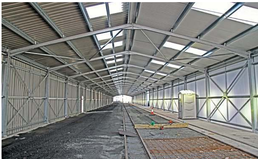
The view along the 400ft length of Vale of Rheidol Railway's newly erected Museum Collection and Heritage Rolling Stock Protection Shed, looking towards Aberystwyth, on February 6. At this stage, two roads had been laid with the concrete floor of that on the right in place. A partition wall is being built along the line of the shallow trench beyond the wooden plank, creating an internal one-road area, which will be heated and accommodate historic stock. The centre road and the third road to be laid to the left (both of which will also receive concrete floors) will house the service fleet of carriages. Behind the photographer is a pit for servicing the underside of carriages. The building will be completed in March. CLIFF THOMAS
