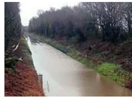
The flooded mainline between Brockenhurst and Bournemouth at Sway.
