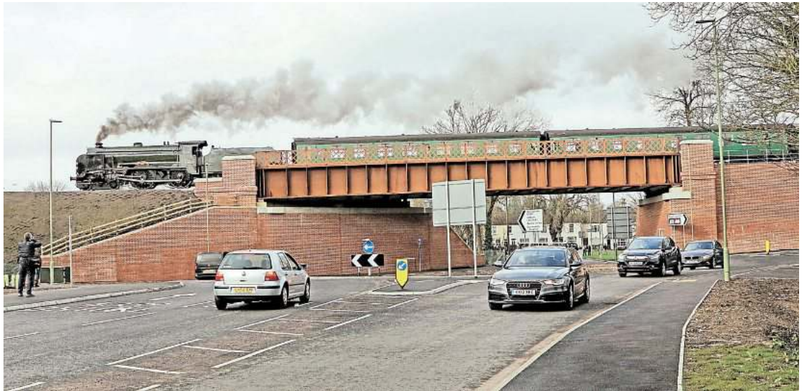
The Mid-Hants Railway's new Bridge 52 is shown to good effect as 'Schools' 4-4-0 No. 30925 Cheltenham makes its first departure out of Alton since the bridge's installation on February 14. PETER ZABEK
