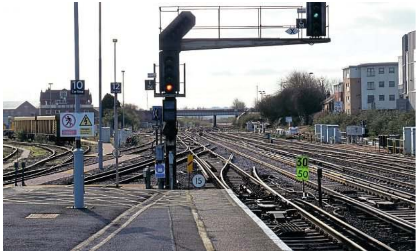
Looking towards Southampton: The partially removed crossover and plain track on the Down Fast line at Eastleigh are clearly visible. This work was carried out as a temporary measure to restore some normality to South Western Main Line services after January 28's derailment at Eastleigh. NETWORK RAIL
