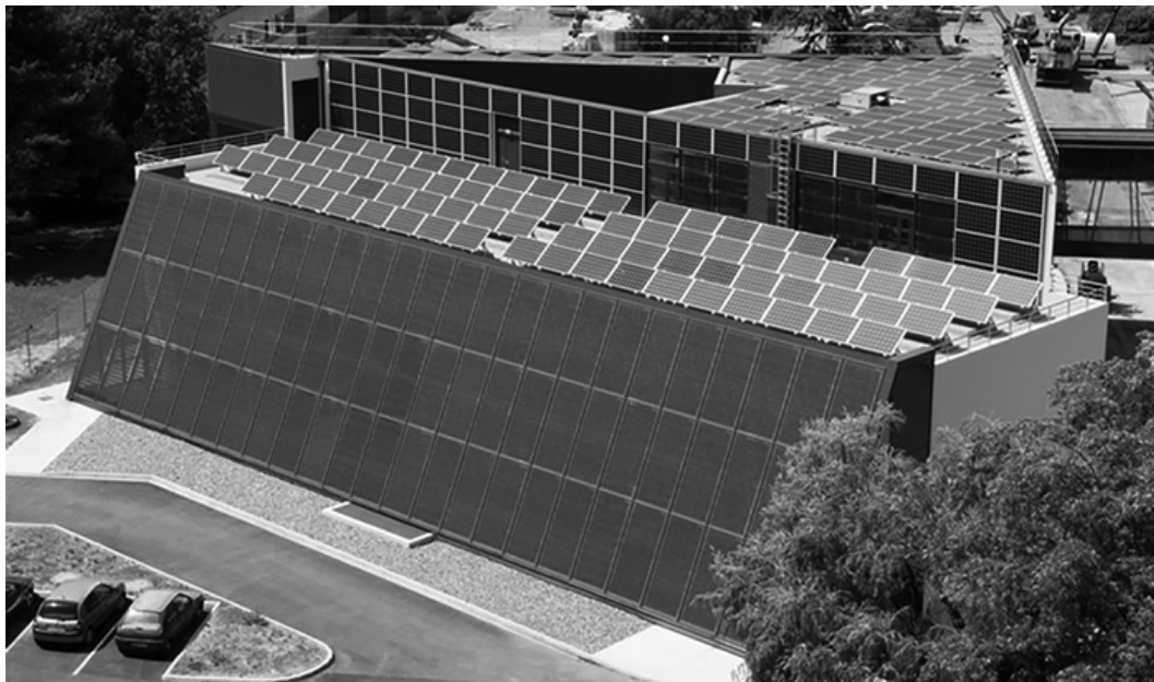
FIGURE 16.1 The Adream building at LAAS-CNRS Toulouse.
