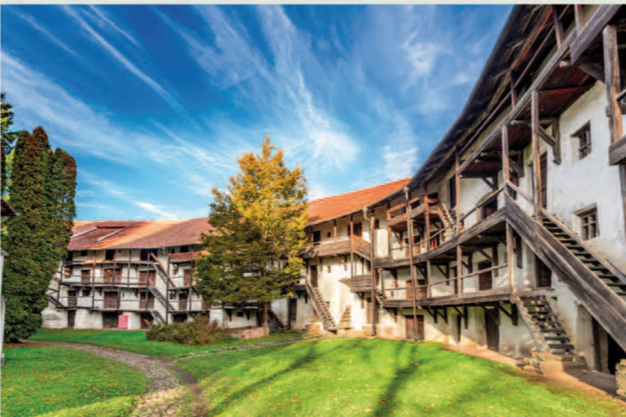
The interior of the curtain wall of Prejmer's fortified church has a total of 272 chambers on three to four levels. These spaces could be accessed through separate entrances, wooden staircases, and walkways.
