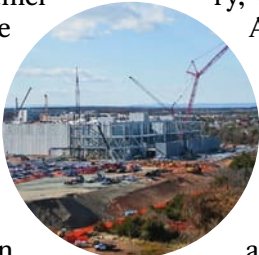
▲ A data center under construction in Ashburn, Va.
